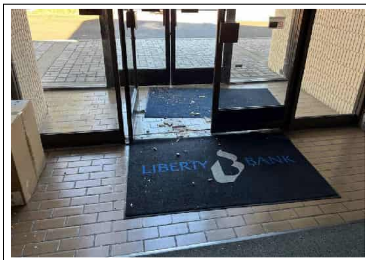
10. View of Tile, Grout, and Mortar Bed
