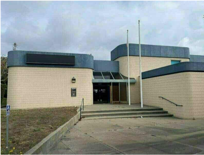
1. South elevation of the building
