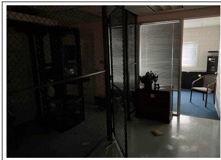
12. View of 2 nd Floor Server Room, VCT Flooring
