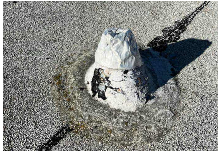
24. View of ACM White/Gray Roof Penetration Mastic
