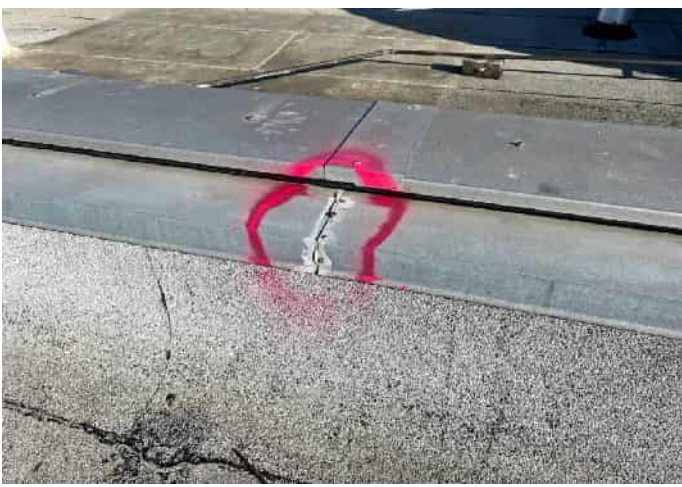
21. View of Parapet and Cap
