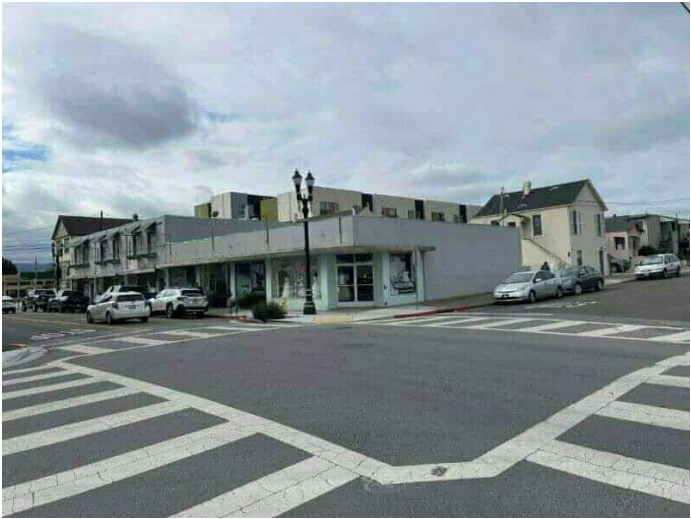
38. Southwest adjoining property
