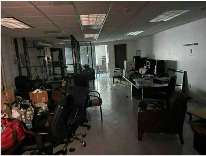
22. Second floor office
