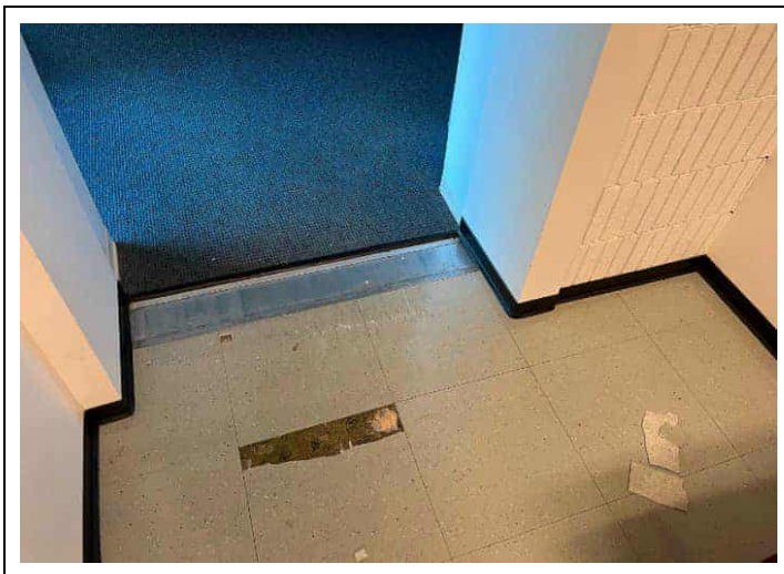
11. View of 2 nd Floor Vinyl Floor Tiles and Cove Base
