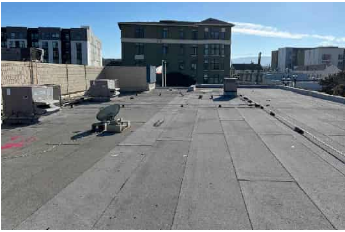
19. View of Lower Roof Area
