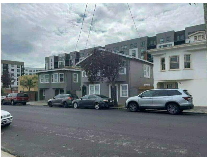
35. Southeast and south adjoining properties
