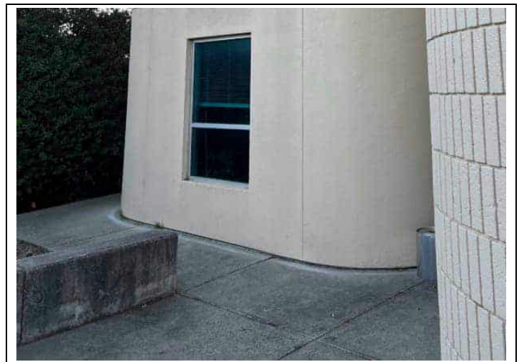
4. View of Typical Window, Exterior Concrete
