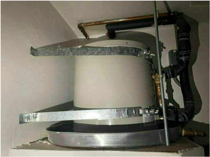
26. Electric water heater
