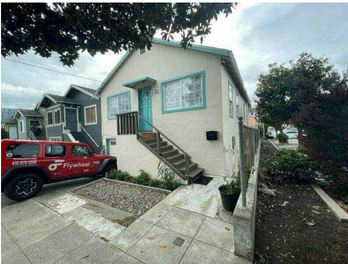
33. East adjoining property
