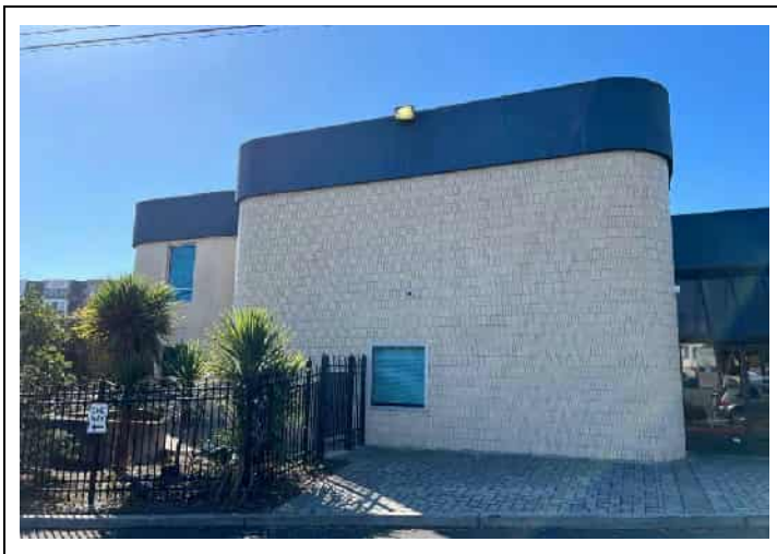
3. View of Masonry Brick Exterior Walls
