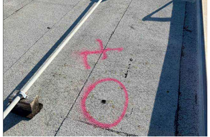
20. View of Main Roof Rolled Roofing
