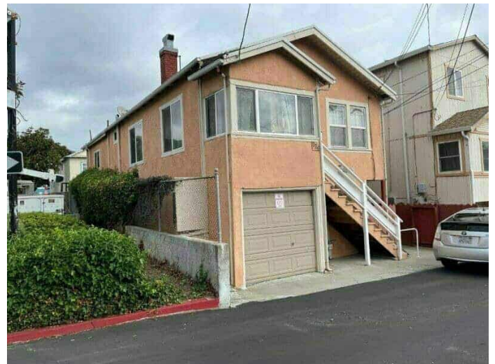
34. East adjoining property
