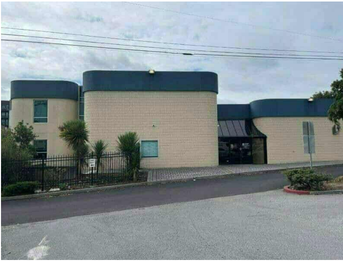
3. North elevation of the building
