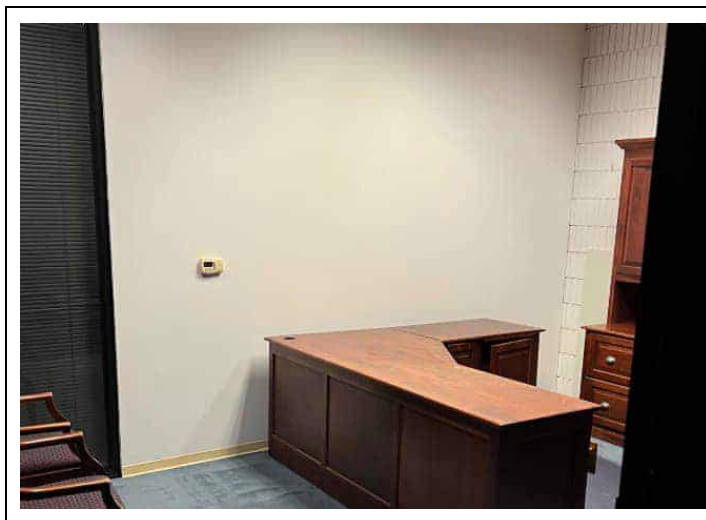
18. View of Office Area w/ Drywall, Cove Base & Carpet
