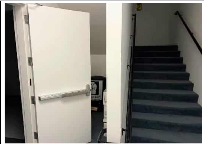
13. View of Carpet on Stairway
