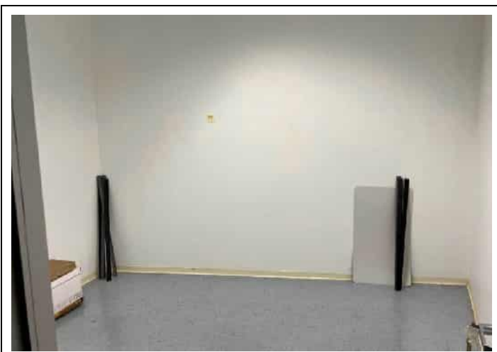
15. View of Storage Area VCT and Cove Base
