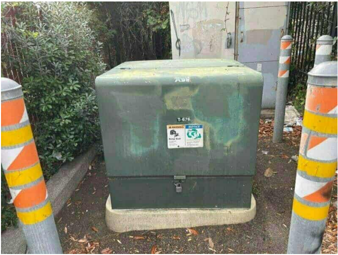
28. Pad-mounted transformer
