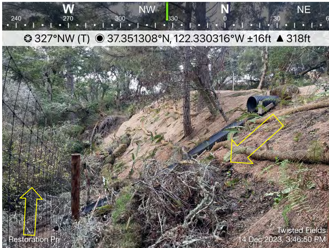
Photo 4. Restoration work area from Pine Tree Gulch.
