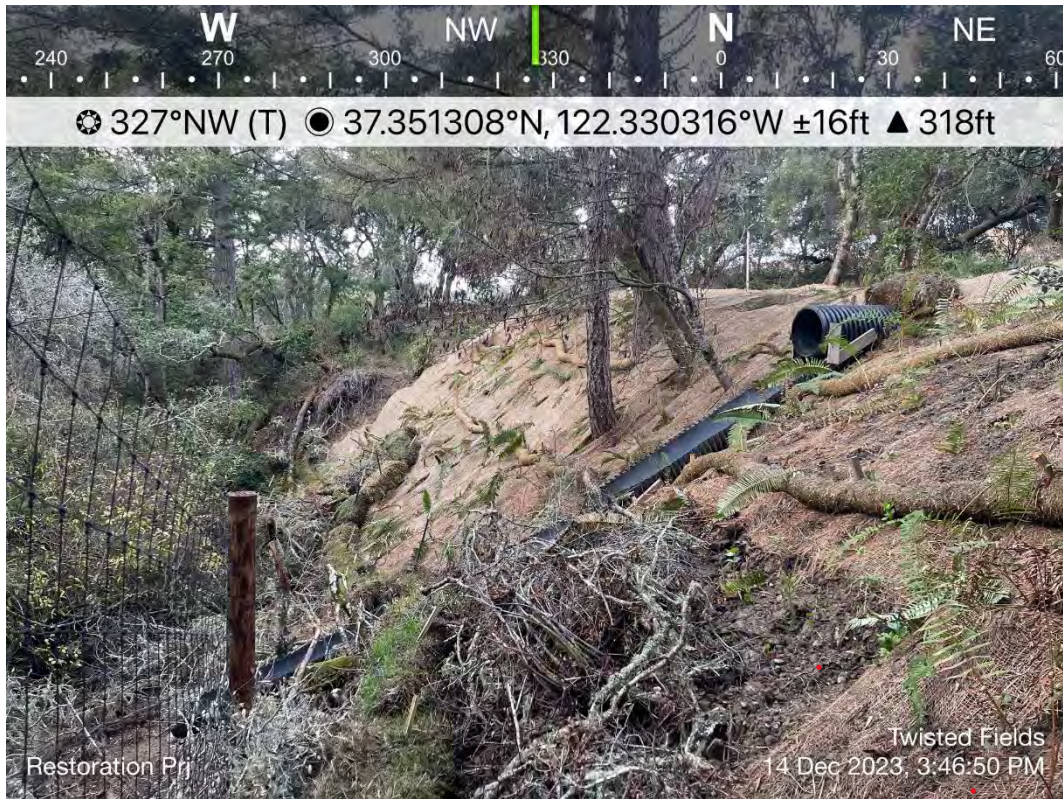
Photo 7. Restoration work area from Pine Tree Gulch.
