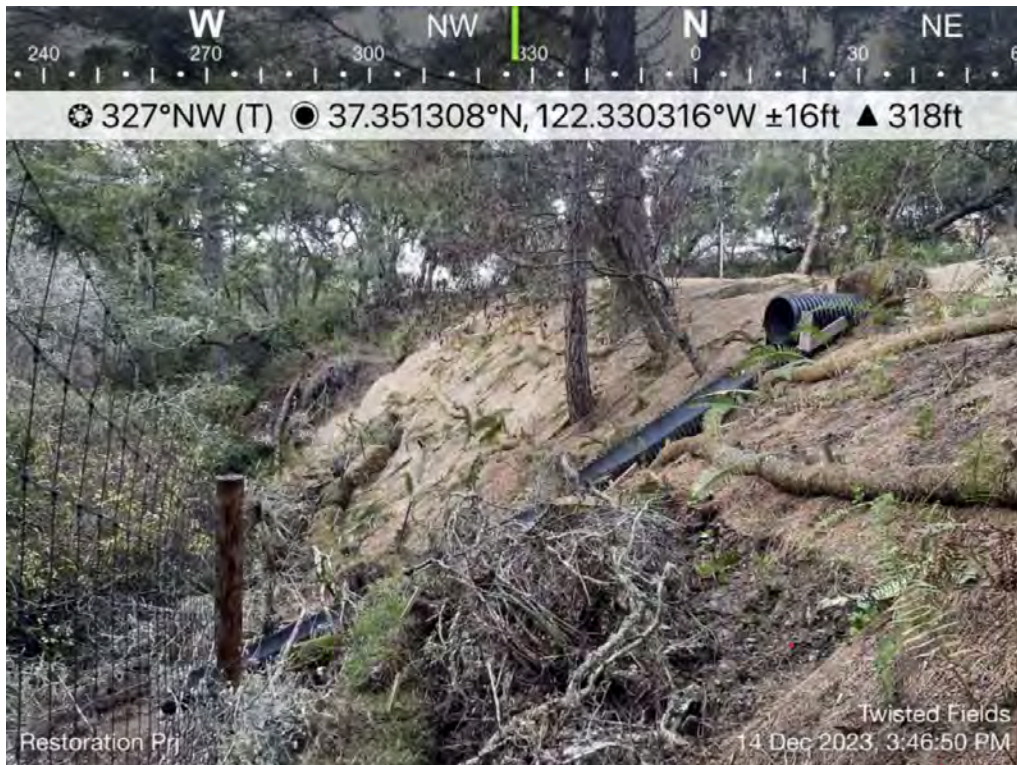
Photo 2. Restoration work area from Pine Tree Gulch.
