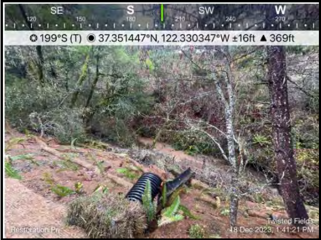
Figure 5 Culvert outfall to Pine Tree Gulch in Restoration Area, December 18, 2023
