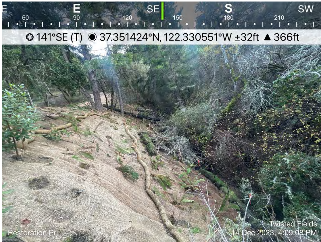
Photo 11. Restoration work area along Pine Tree Gulch.
