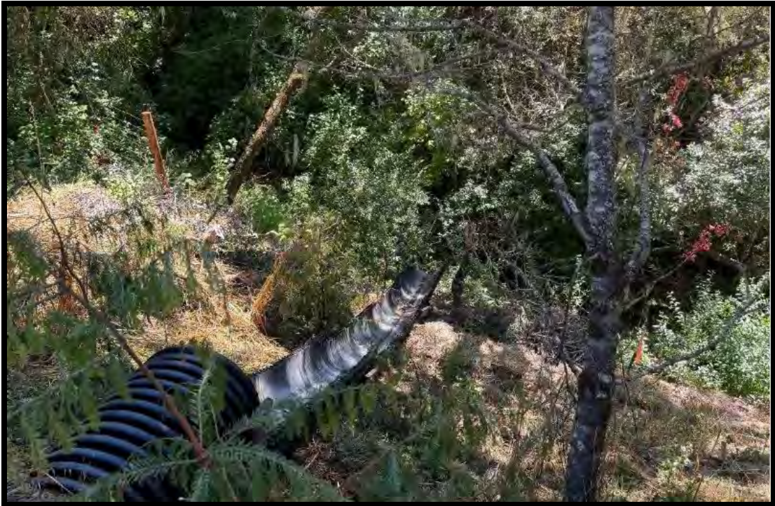
Figure 6 August 2024 picture with BMP Measures installed and increased vegetation cover by 20-30%
