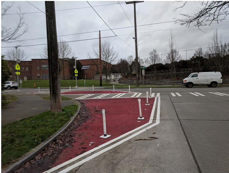
Painted Curb Extension (Bulb-Out) with Delineators
