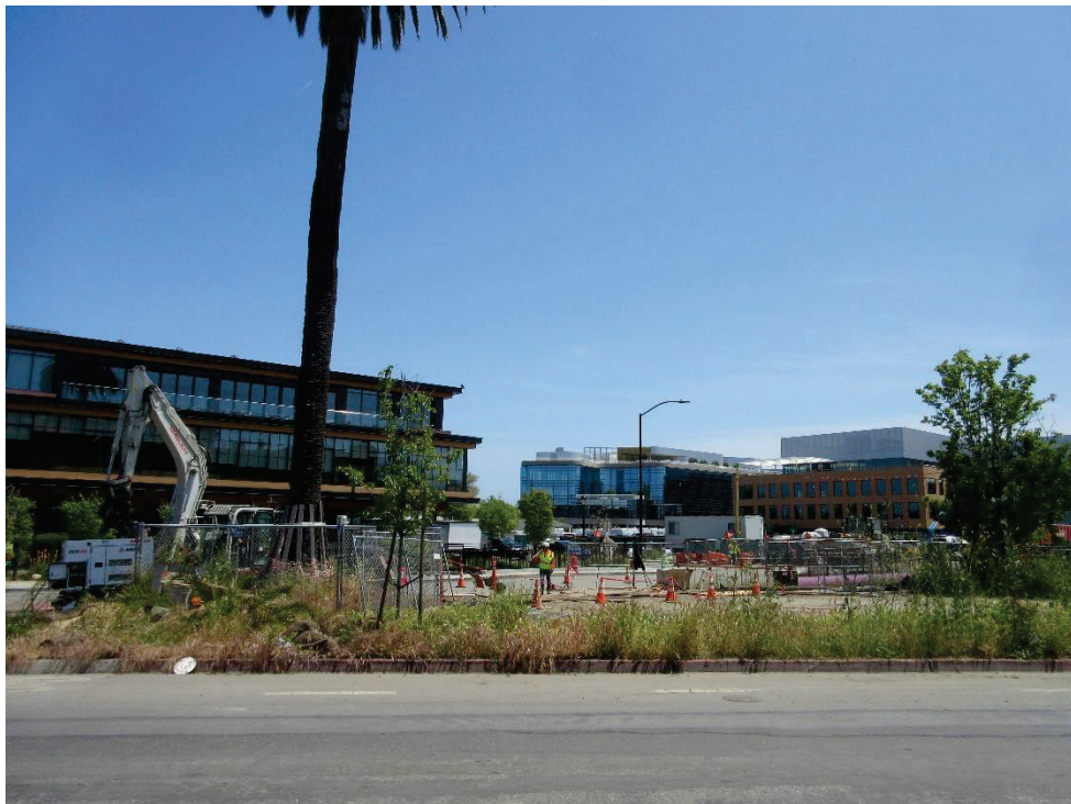
VIEW FROM MAPLE STREET LOOKING SOUTHEAST
