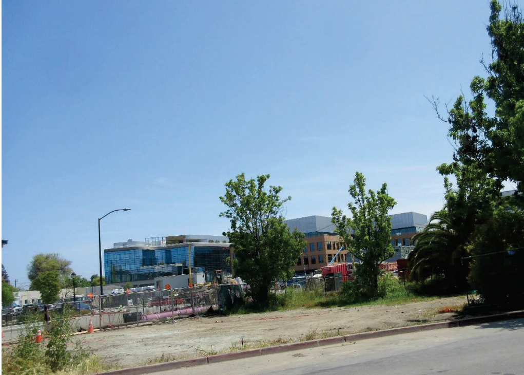
ON-SITE VIEW LOOKING SOUTHEAST
