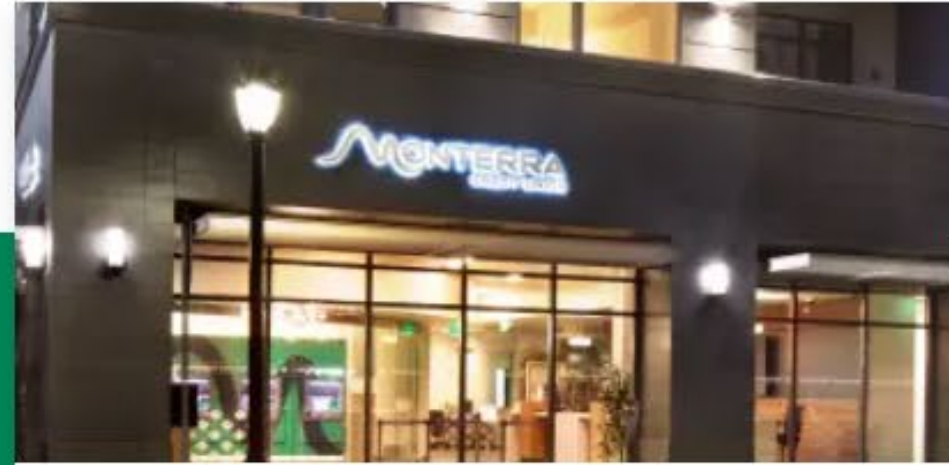
Redwood City Main Branch
