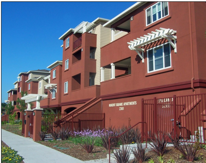
Nugent Square Apartments—East Palo Alto @ County of San Mateo
