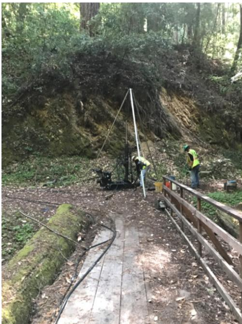
Photograph 1. B-1, east of bridge, drilled with a portable rig
