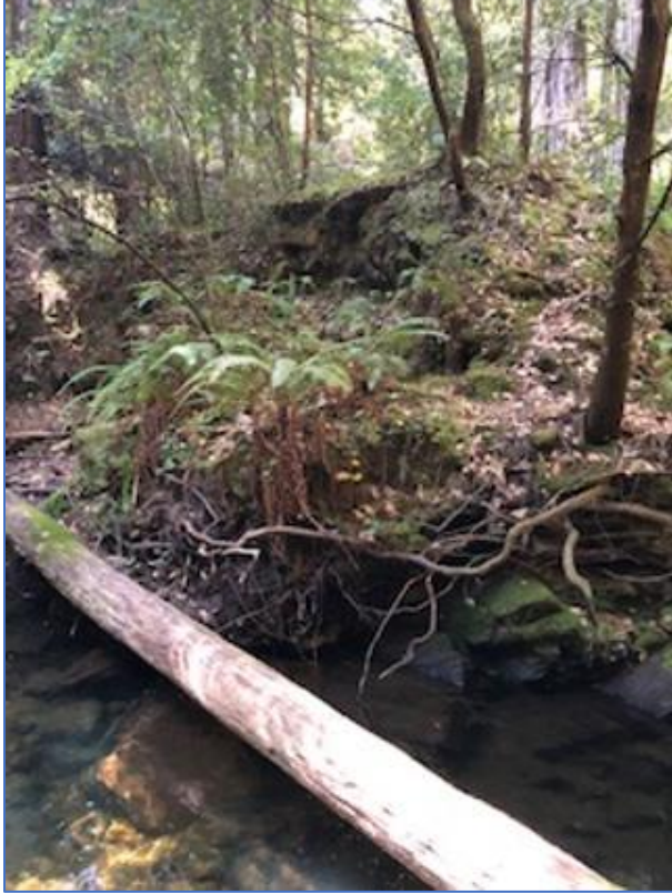
View 9. View upstream at the southeast bank of the upper bridge crossing.
