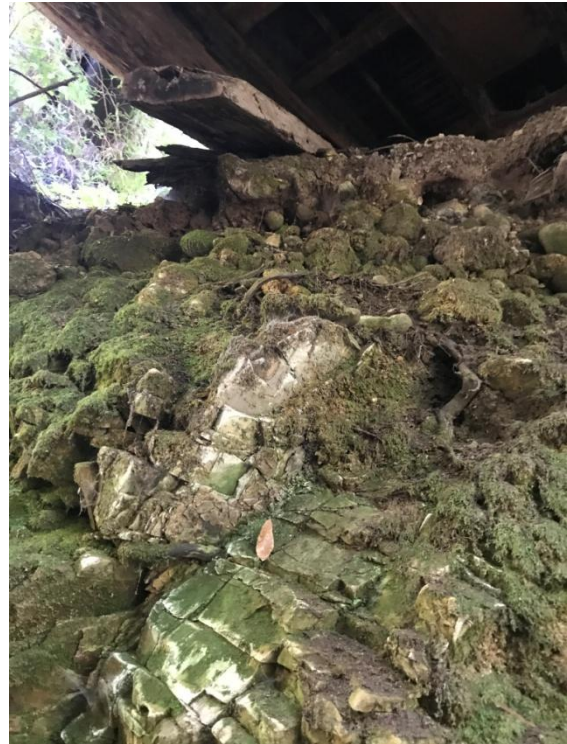
Photograph 4. Bedrock exposed beneath existing bridge at proposed Bridge Crossing 2.
