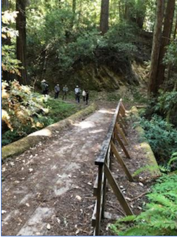
View 1. View to east of existing bridge crossing of Peters Creek.
