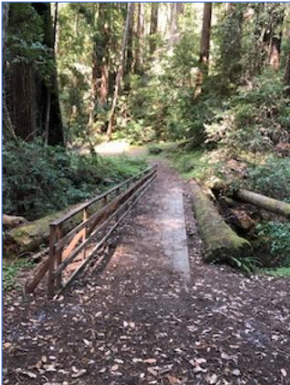
View 2. View to the west of existing bridge.
