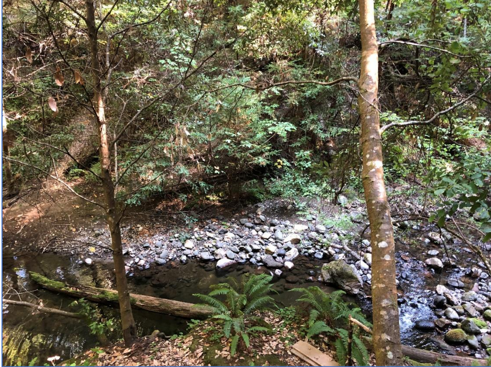
View 7. View of upper crossing from southeast bank, near new bridge footing.
