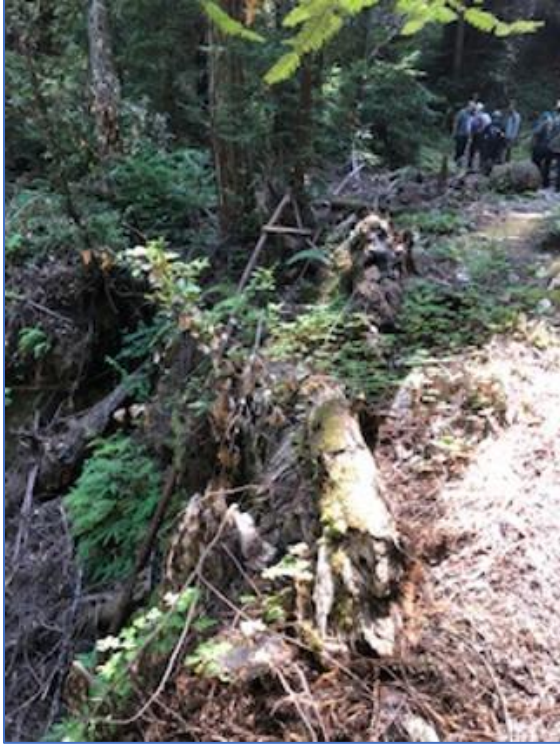
View 5. View of south bank to be repaired and stabilized.
