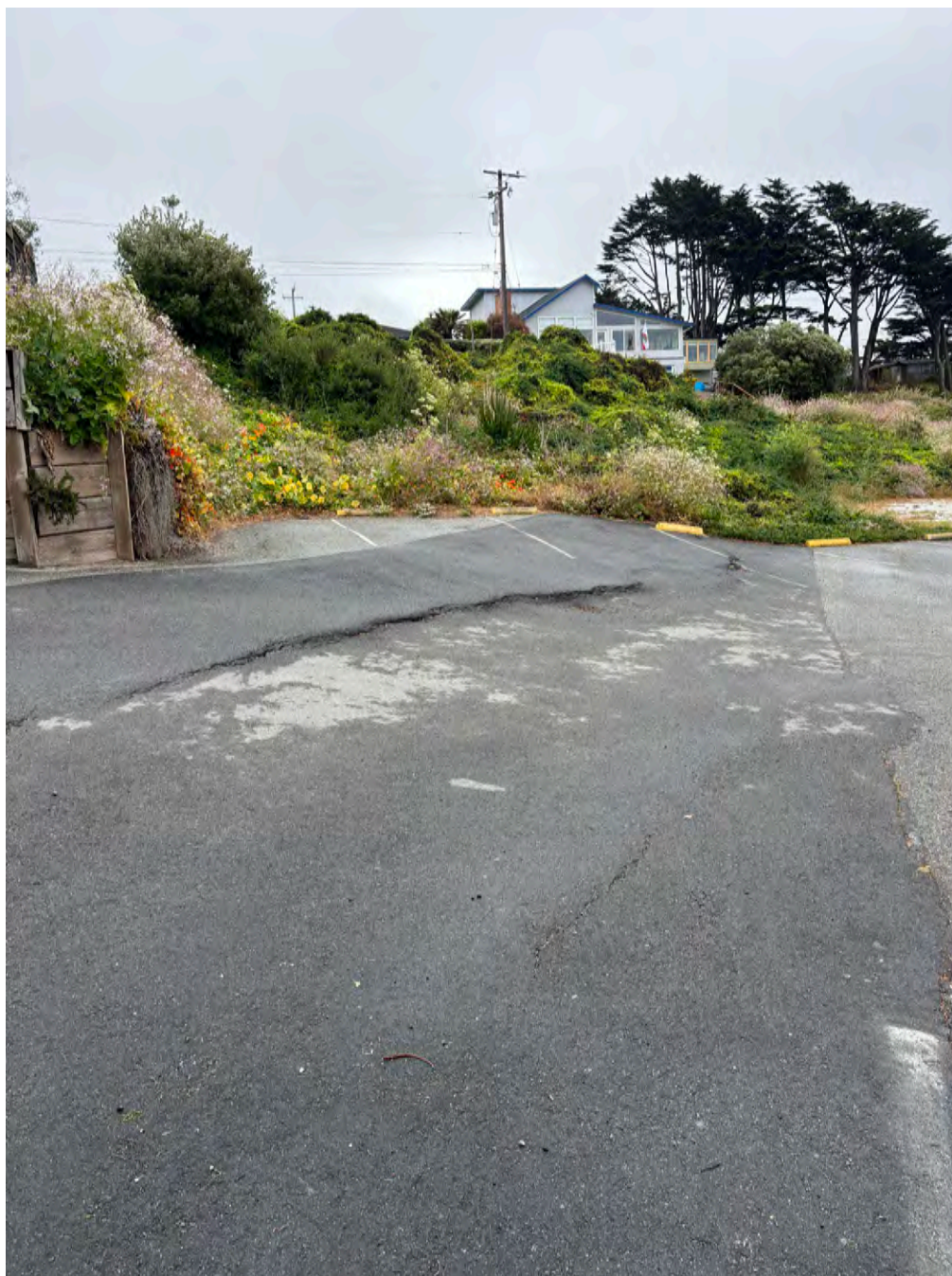
Photo 3: Scarp in Moss Beach Distillery parking lot, east of the restaurant. Photo taken facing southeast. Date of photo: June 25, 2025.
