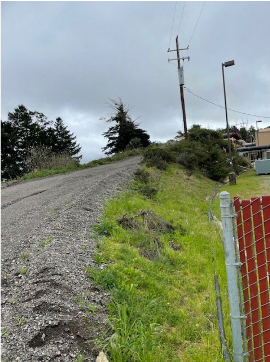
Figure 11 – Landfill Perimeter Road on the southern side of the facility.
