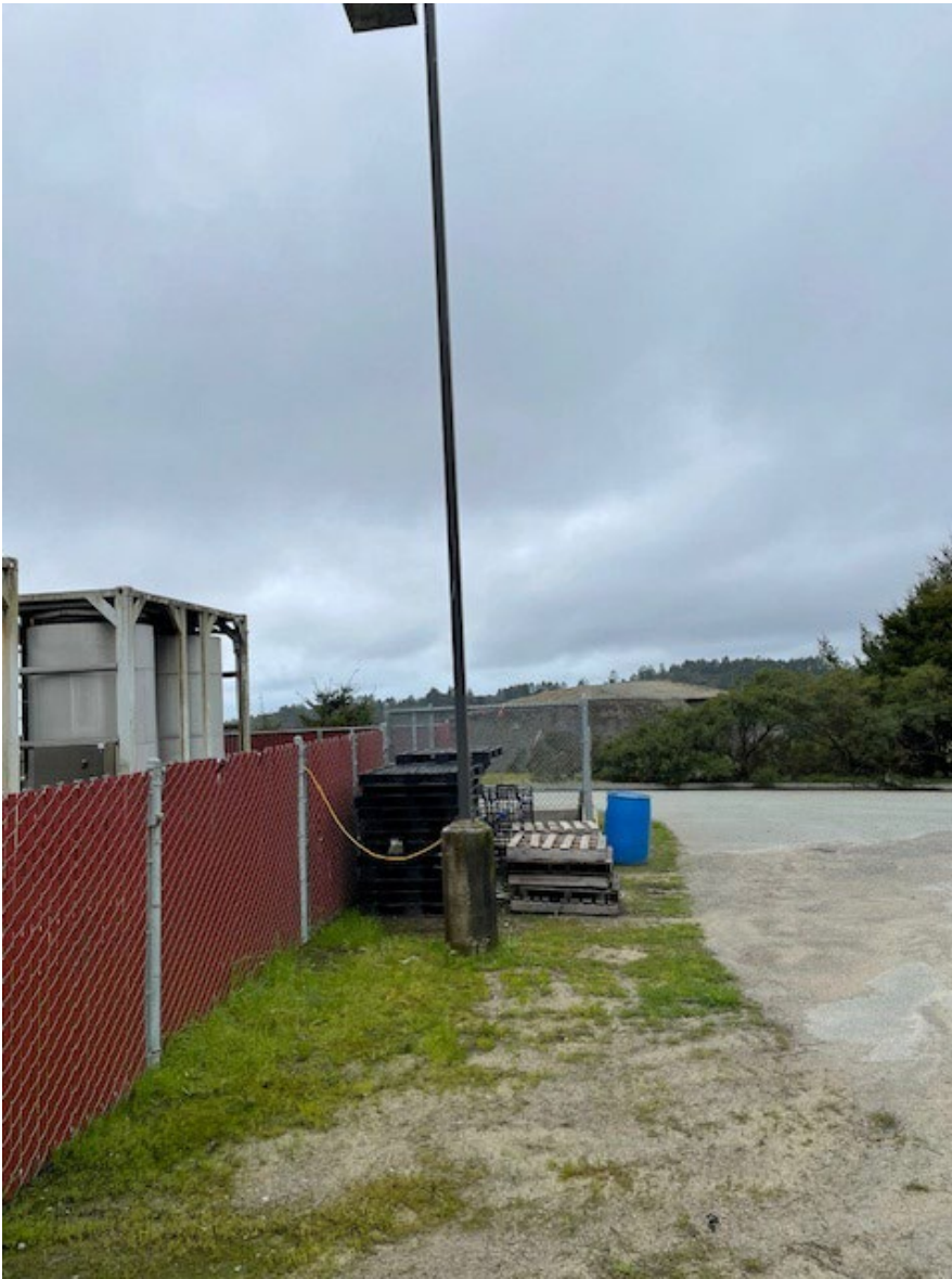
Figure 10 - Northern Area of the facility. Equipment will be installed in the area where the pallets are stored. The area covered in gravel is the Fire Truck turn around area.
