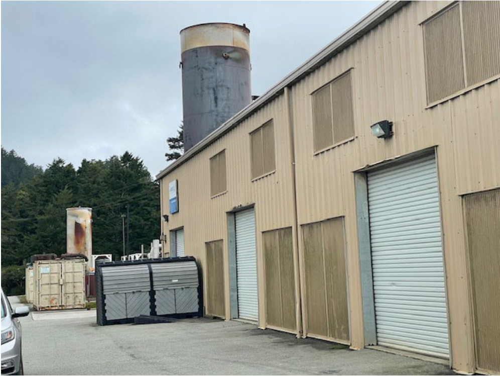
Figure 3 - Ameresco Co-generation Facility at Ox Mountain
