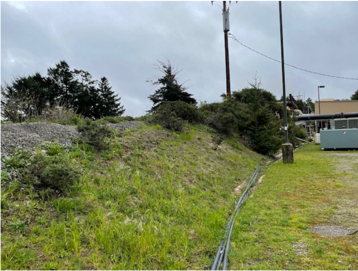
Figure 9 - Proposed Northern expansion area. Ameresco plans to cut into the slope and install a retaining wall for area to install additional equipment.
