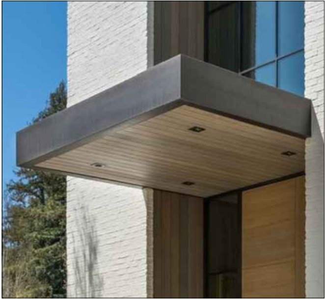
HORIZONTAL CANTILEVERED ROOF COVER AT ENTRY
