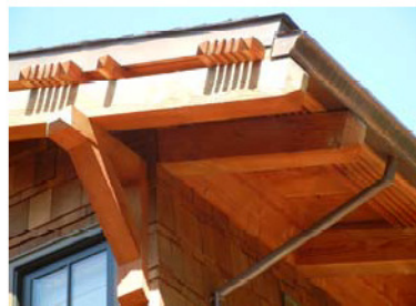
Building with copper flashing, gutter and drainpipe.
