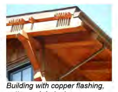
Building with copper flashing, gutter and drainpipe.
