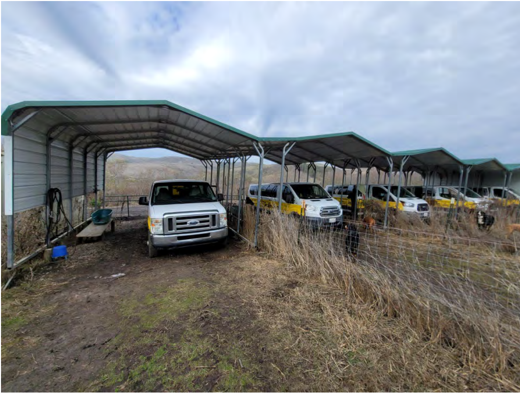
Staging Area View 1: Five aluminum carports being used as staging area for dog hiking operation
