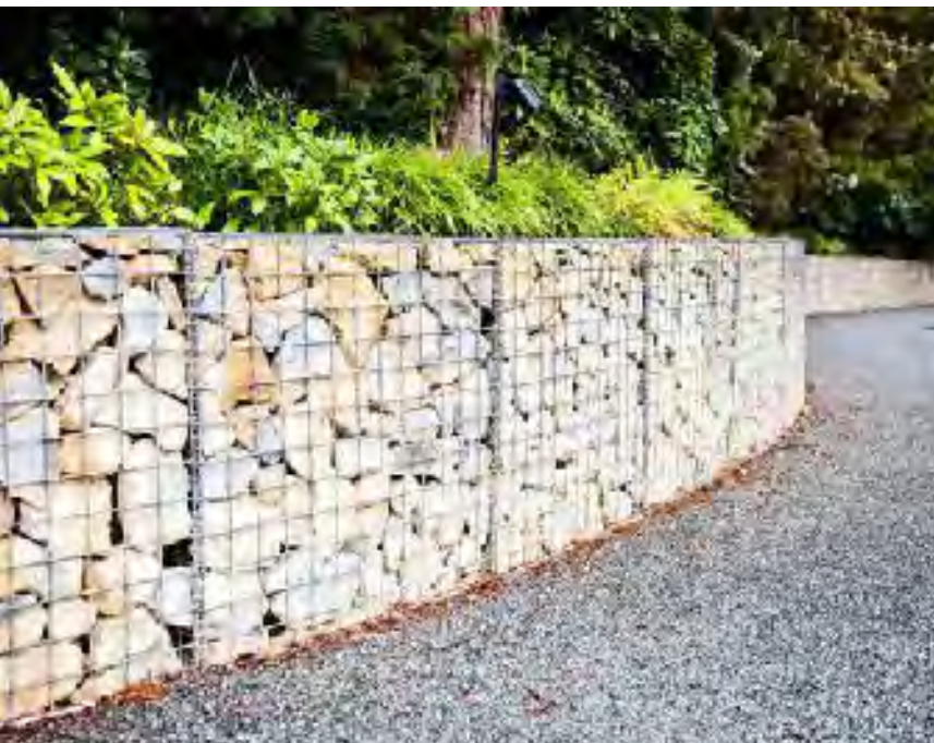
TYPICAL GABION WALLS & GABION BENCHES
