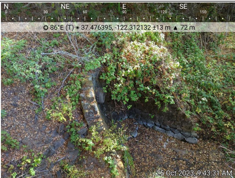
Photo 8. The outfall of the preexisting drainage system. The scope of work proposes tying the new drainage system in approximately 100 feet up from the headwall to avoid encroaching into CDFW jurisdiction.
