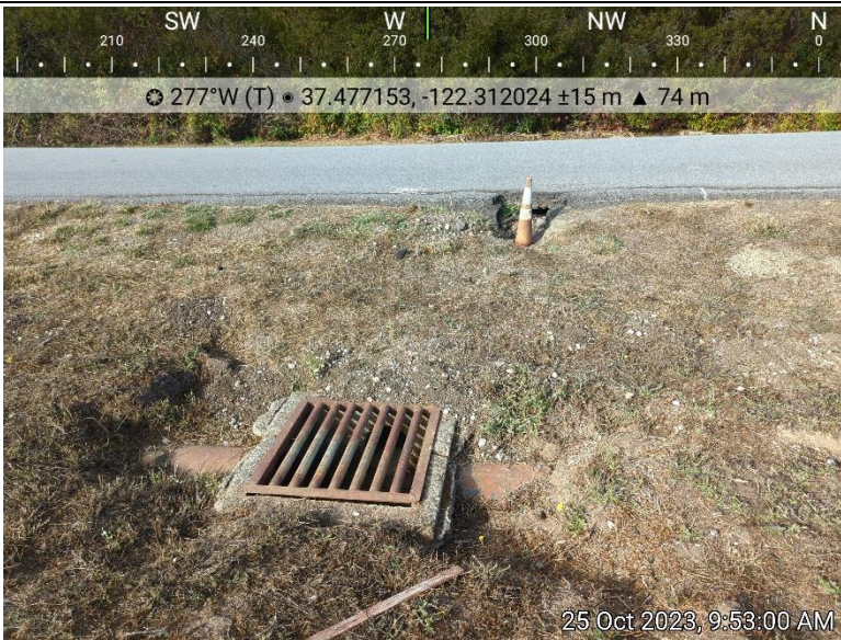
Photo 5. The preexisting drainage system along the access road. The drainage is not currently functional and will be removed and replaced in the current scope of work.
