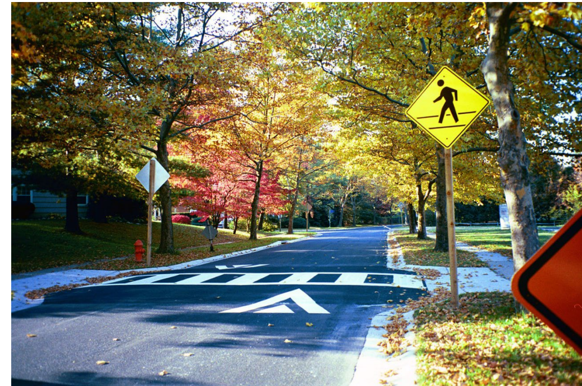
Raised Pedestrian Crossing
