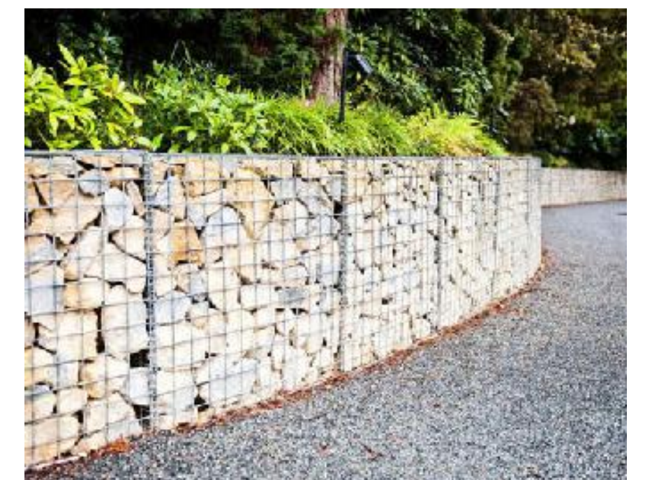
TYPICAL GABION WALLS & GABION BENCHES
