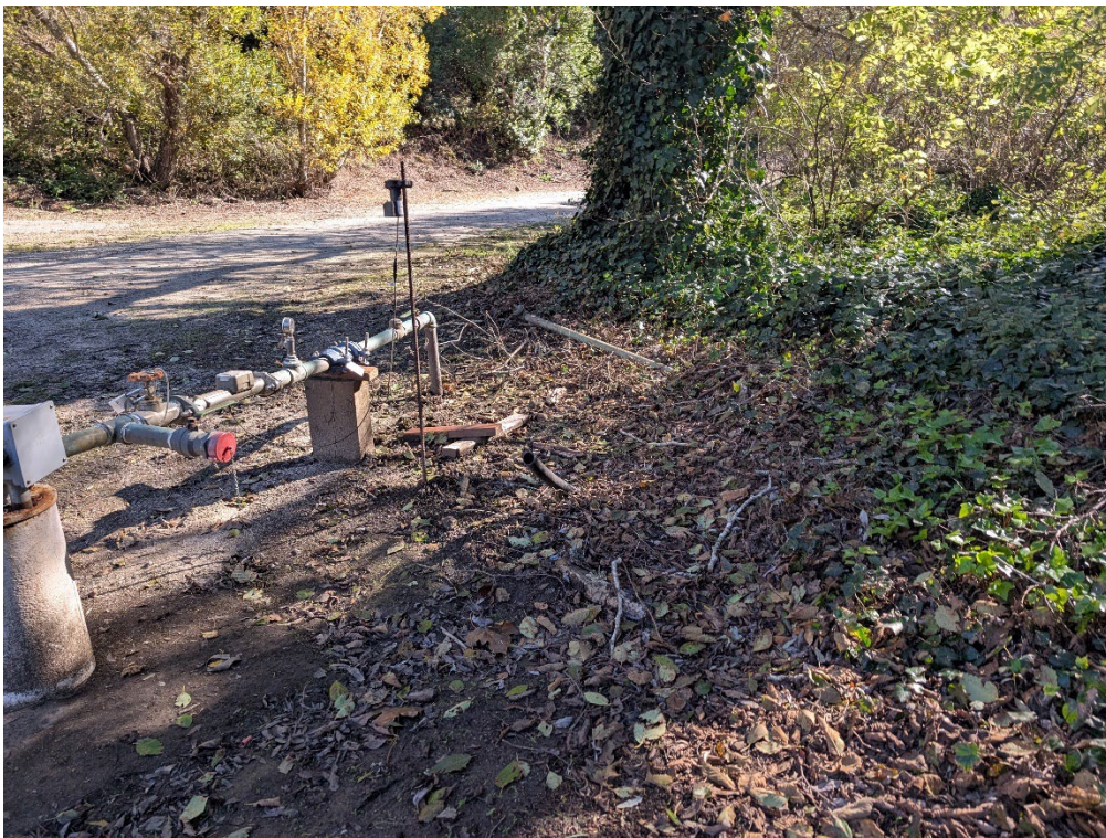
Photo 14. Existing Well and Pilarcitos Creek Road
