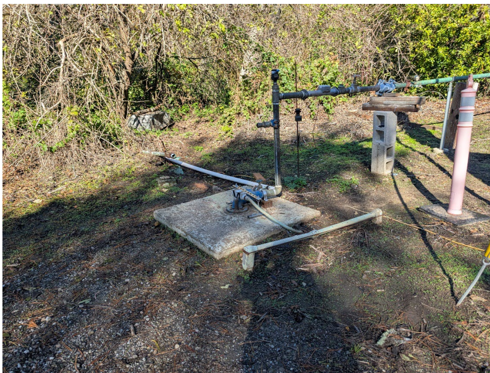
Photo 16. Existing Wells, Pilarcitos Wellfield, and adjacent vegetation
