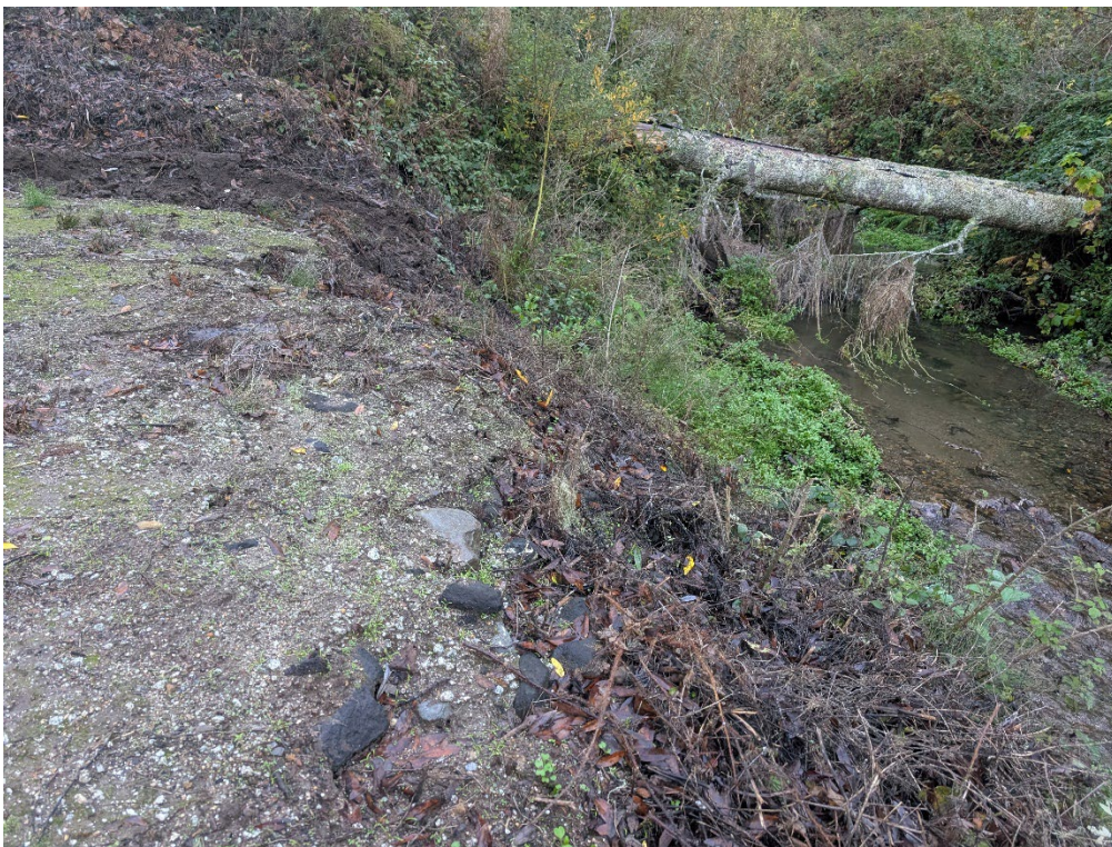
Photo 6. Pilarcitos Creek and Creek Bank
