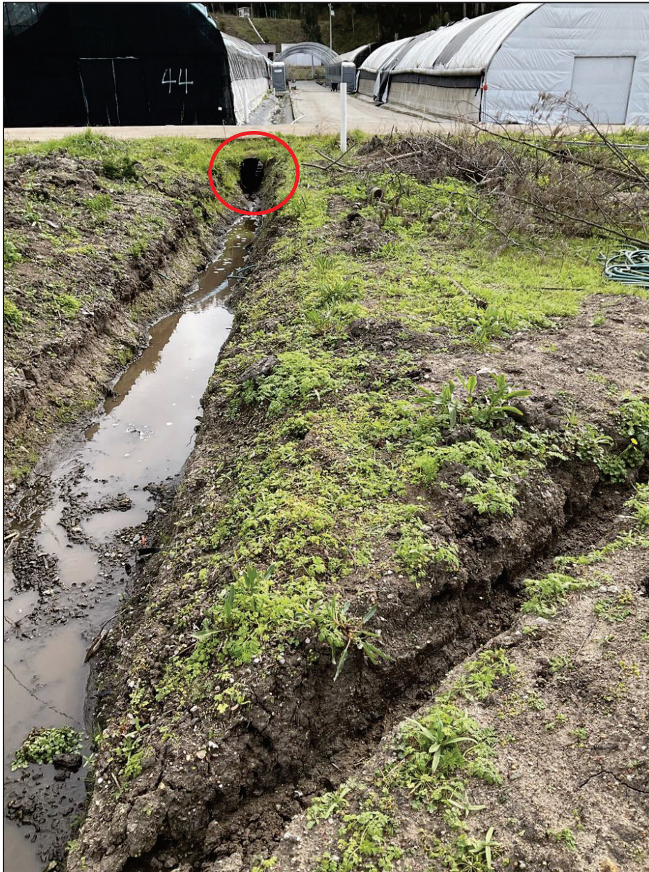
Figure 10. A 26-inch corrugated metal pipe (red circle, SC-1) marks the transition to a modified tributary that flows to Pilarcitos Creek.
