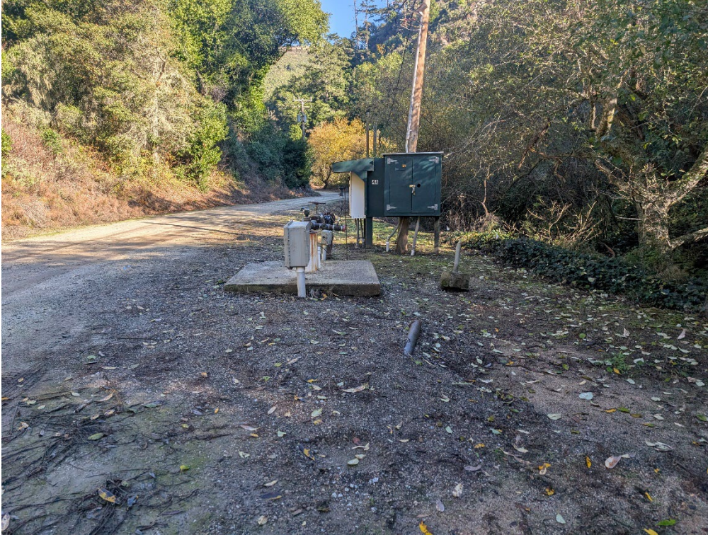
Photo 7. Existing Well, Wellfield and Pilarcitos Creek Road
