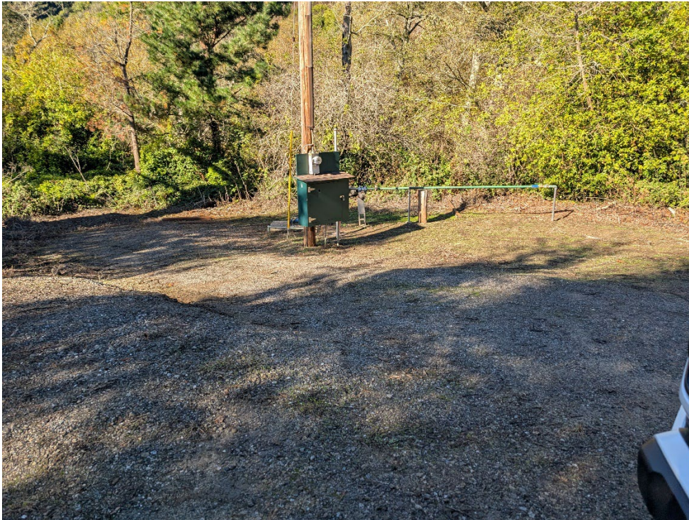
Photo 15. Pilarcitos Creek Road and Pilarcitos Wellfield
