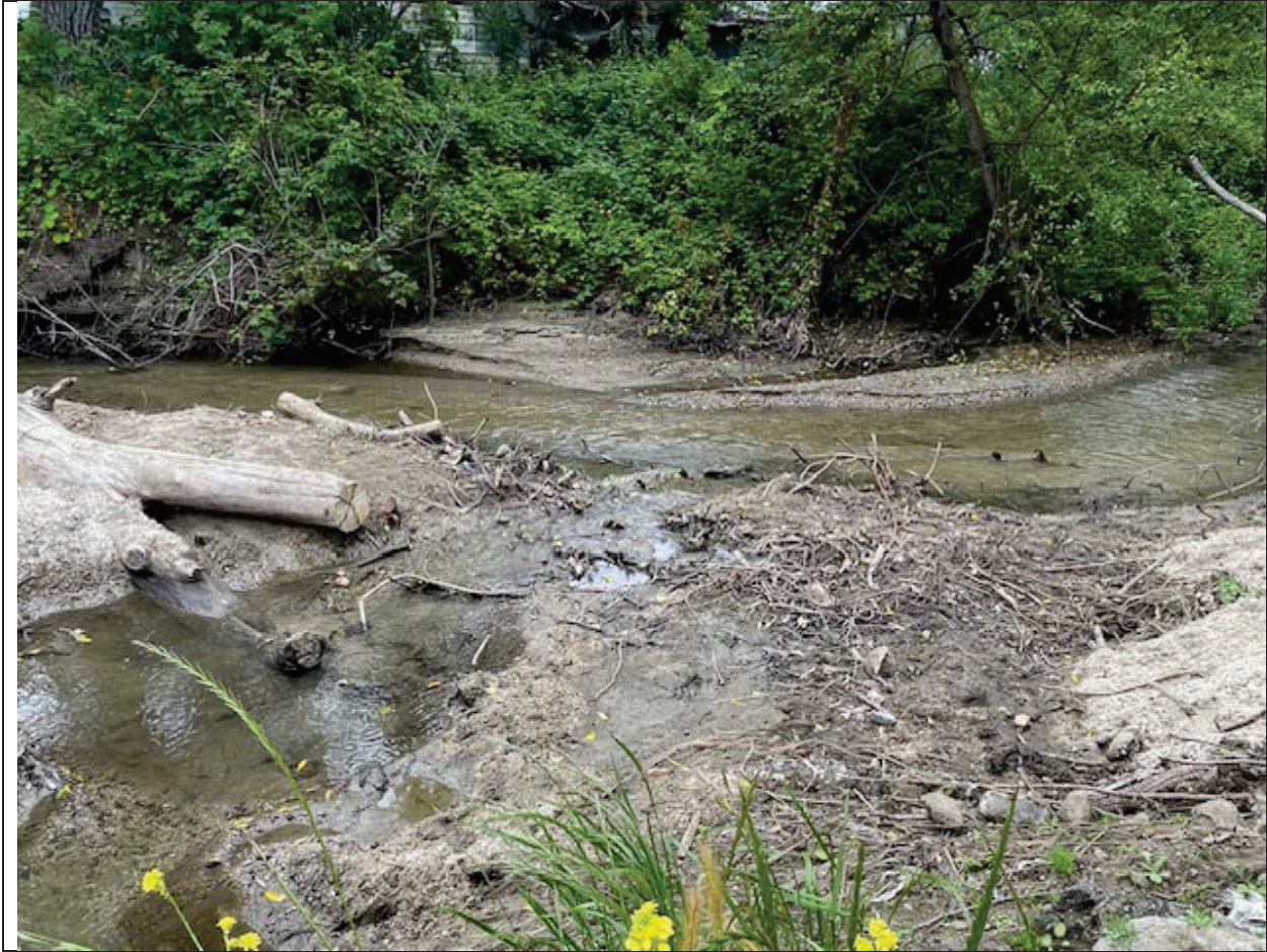
Photo 6. Action 4 – Diversion structure removed as of June 7, 2023
