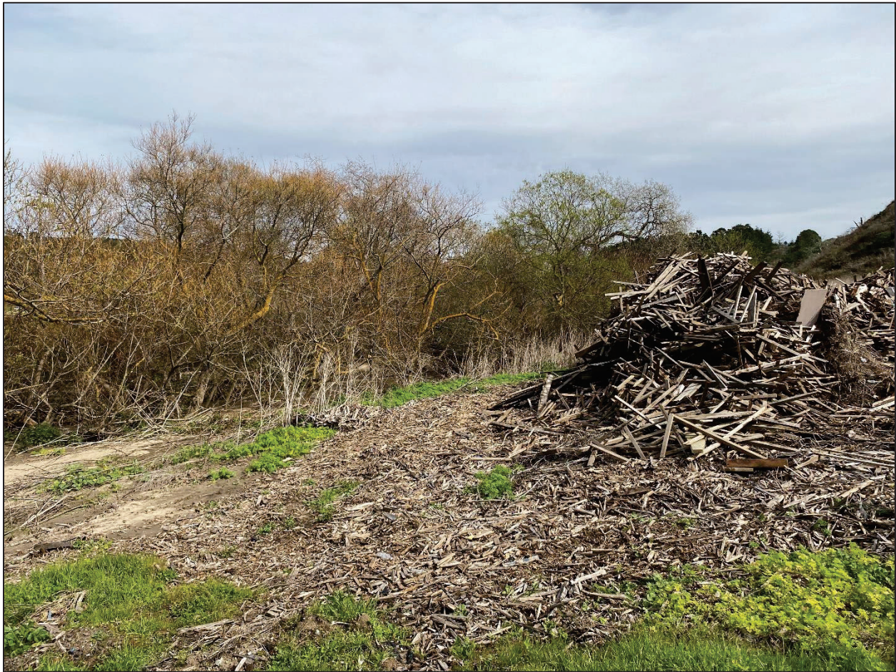
Figure 12. Wooden debris from a demolished building at PP-3 within 150 feet of Pilarcitos Creek.
