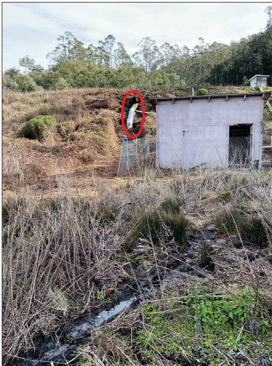
Figure 8. An existing earthen dam built on-top of an unnamed tributary prevents water from flowing downstream until the water surface level in the reservoir (WSt-2) reaches the culvert spillway (circled in red).
