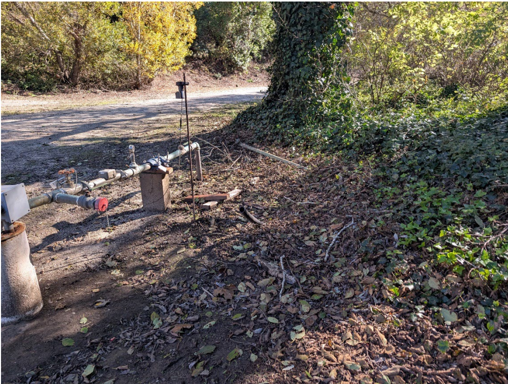
Photo 14. Existing Well and Pilarcitos Creek Road
