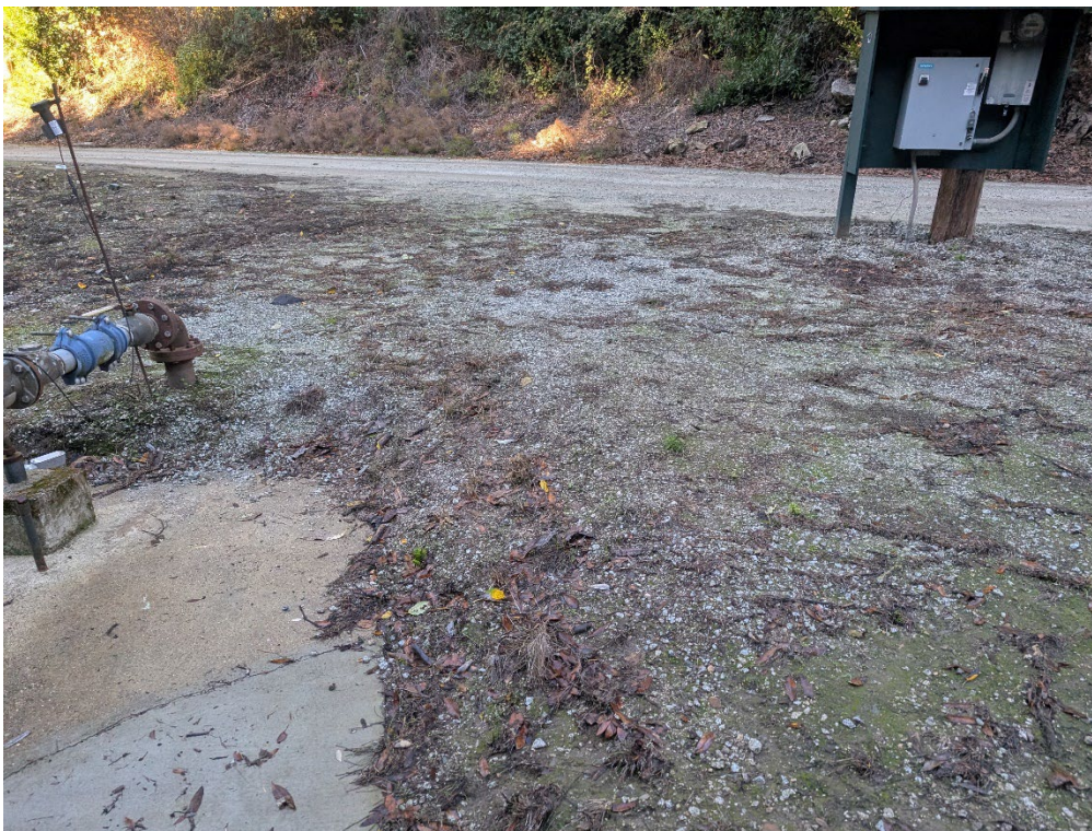
Photo 4. Existing Well, Pilarcitos Creek Wellfield, Pilarcitos Creek Road
