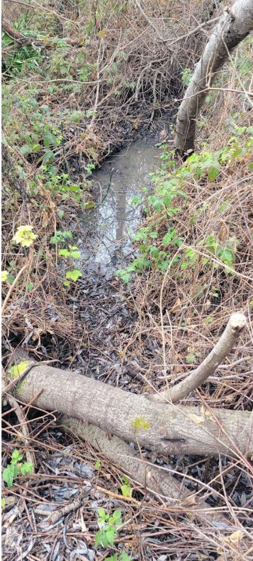
Left – Channel built by downhill property owners on Lacasia lot, directing water away from adjacent property and creek. February 2025, not a wet year.
