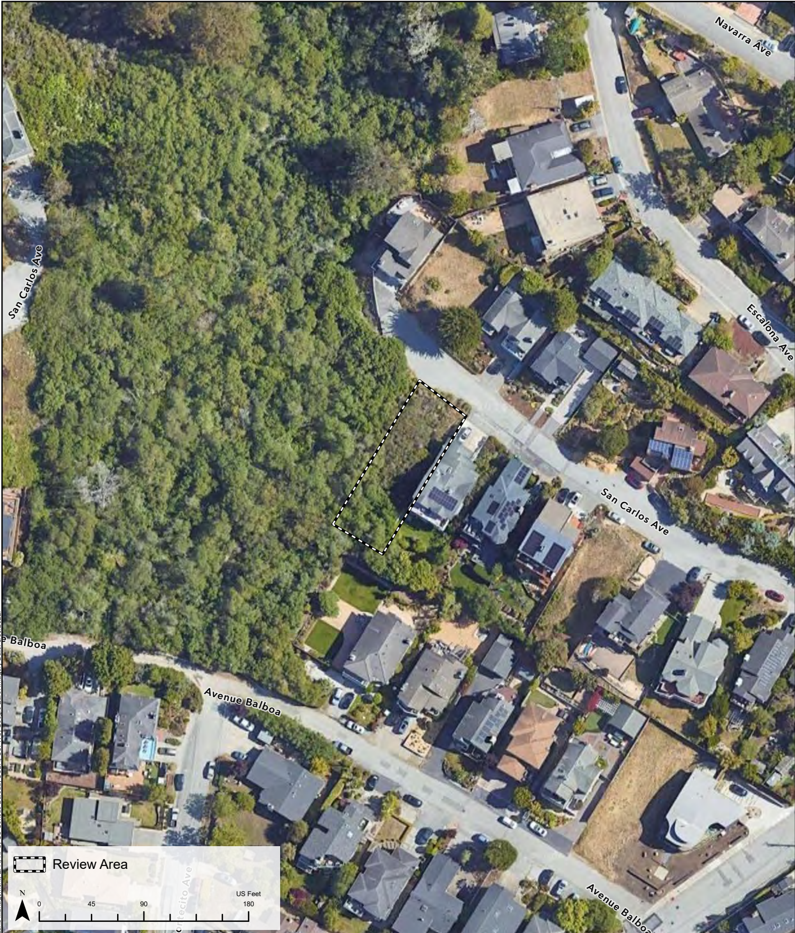
Figure 3. Aerial Image of the Review Area Proposed Single-Family Residence Project 779 San Carlos Avenue, El Granada, San Mateo County
