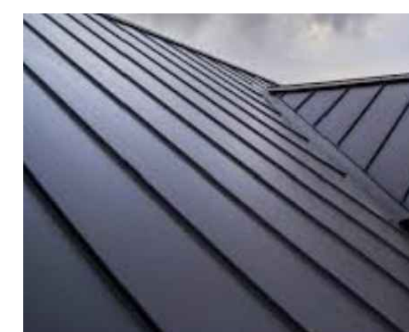
GALVANIZED METAL ROOF FOR DORMER ONLY
