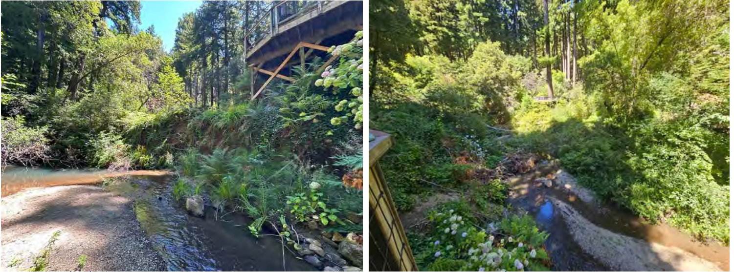
PHOTO 4 (LEFT). VIEW OF EAST STREAMBANK PHOTO TAKEN FROM MID-STREAM, ANGLED UPSTREAM. PROPERTY OWNER'S DECK CAN BE SEEN IN TOP RIGHT.
