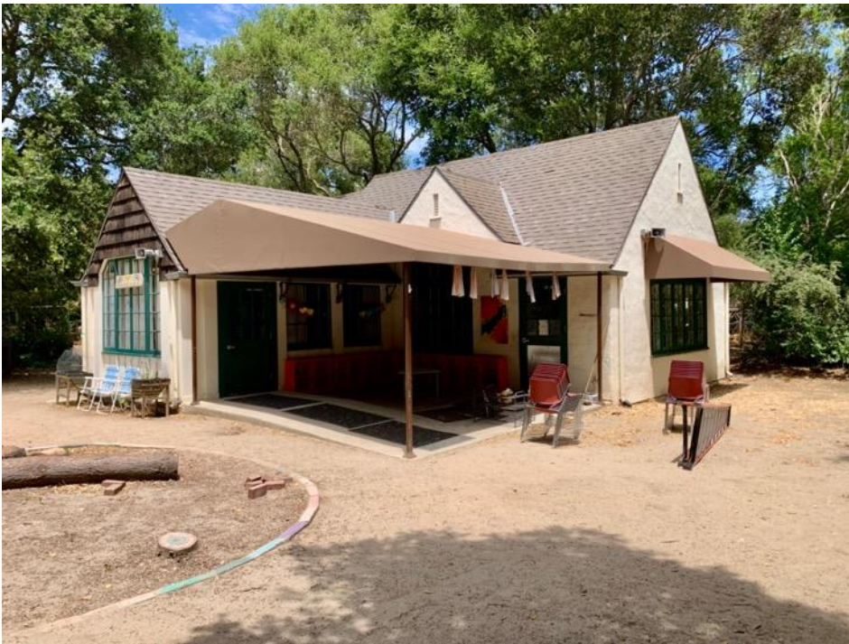
Figure 3. South and west elevations including exterior covered patio, view looking northeast
