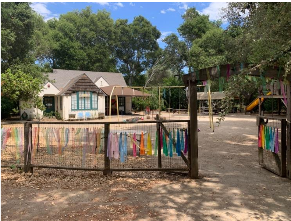
Figure 17. Fenced entry to Building 1 along Peninsula Way, view looking northeast
