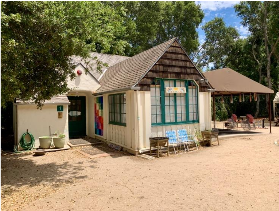
Figure 8. Partial west and north elevations showing primary entry, view looking generally southeast
