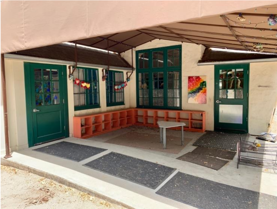
Figure 4. Detail view of covered patio area, view looking northeast
