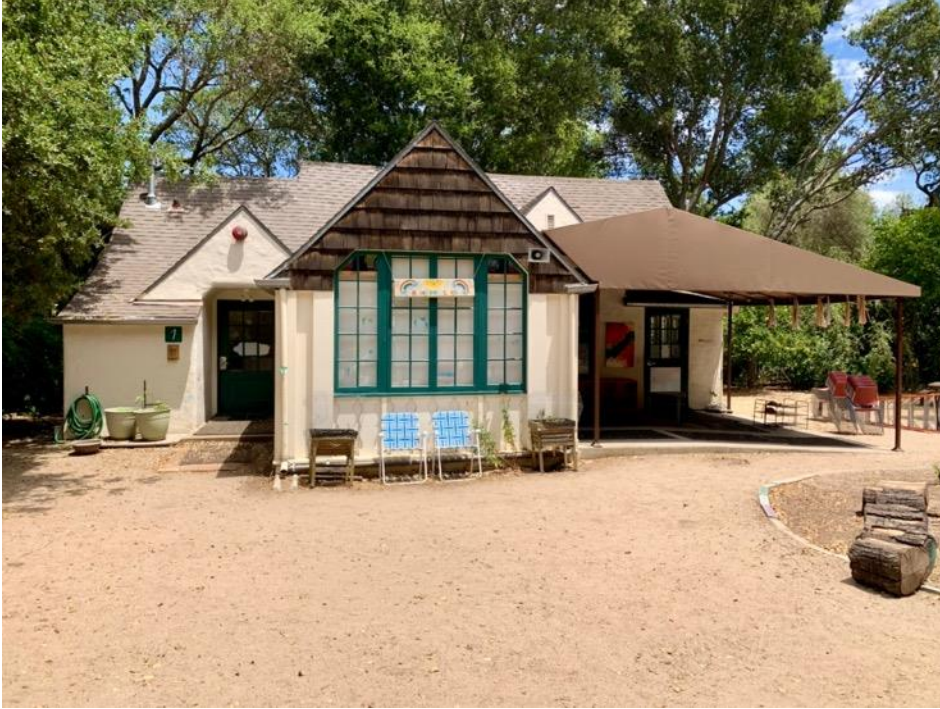
Figure 2. West elevation, view looking east
