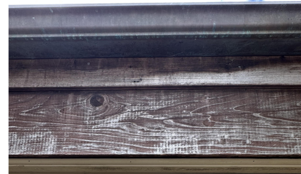
(E) GUTTER MATERIAL: - COPPER
