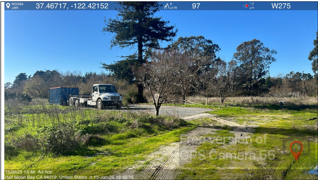
Photo 1. Action 1 – mobile home (R1, R2) removal
