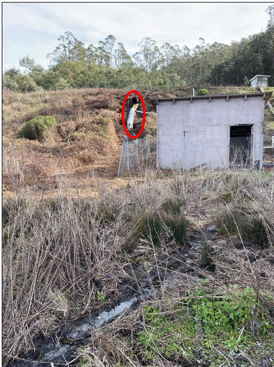
Figure 8. An existing earthen dam built on-top of an unnamed tributary prevents water from flowing downstream until the water surface level in the reservoir (WSt-2) reaches the culvert spillway (circled in red).
