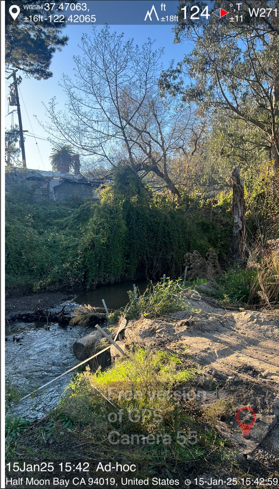
Photo 5. Action 4 – diversion structure removal location.
