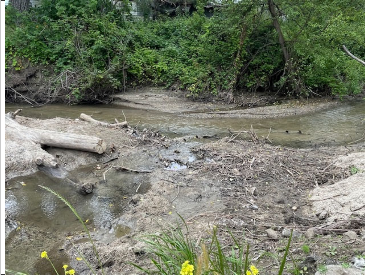
Photo 6. Action 4 – Diversion structure removed as of June 7, 2023
