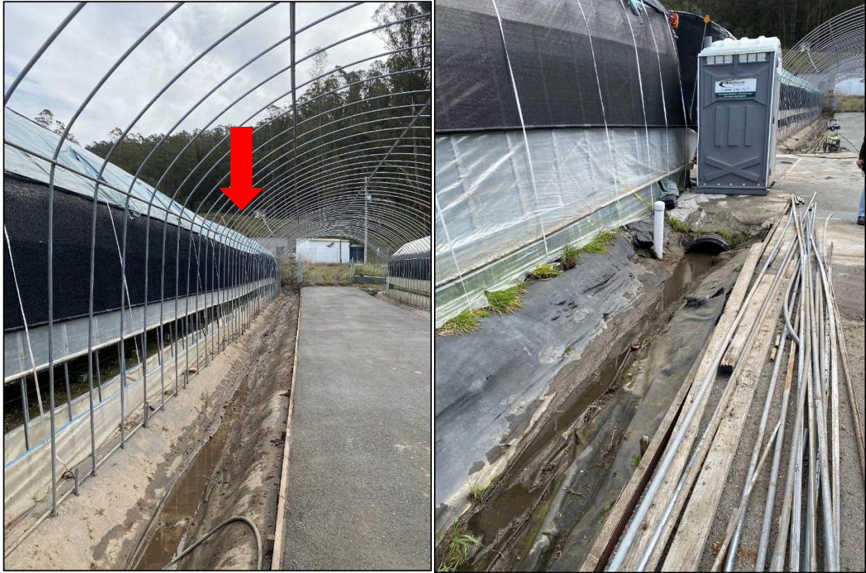
Figure 9. A concrete and geotextile-lined modified tributary adjacent to a mushroom building (left and right picture, PL-1). The reservoir embankment is visible in the background (red arrow in left picture).
