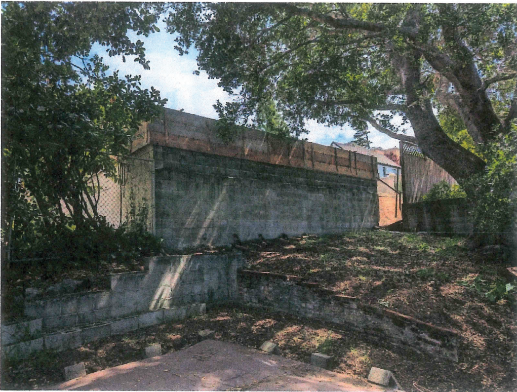
Photo 1 – Retaining wall at property line
