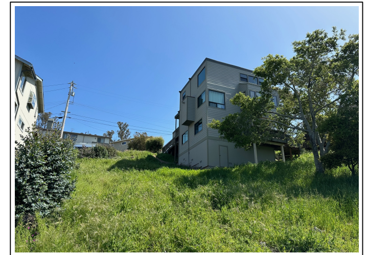
VIEW FROM THE REAR OF THE PROPERTY
