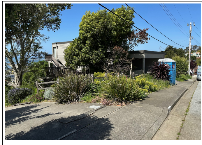
EAST VIEW FROM THE STREET: LEFT SIDE OF PROPERTY
