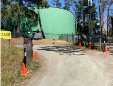
Fence Pump & hydrant.jpg 194K
