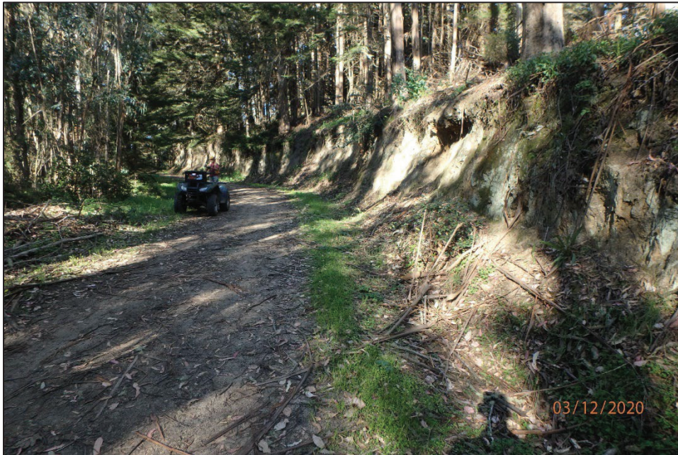
Figure 1: View of a typical road cutbank along a midslope road within Quarry Park. The A horizon within the soil profile, weathered granitic bedrock, and deposit of sandy soil eroded from the cutbank can be identified in the photograph.
