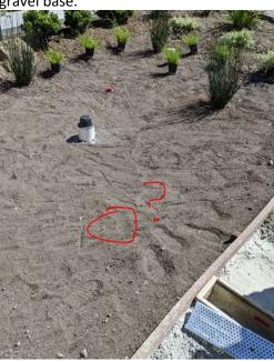
2. There is an extra inlet pipe on each of the side planters – please confirm what this inlet is. If it is a subdrain/inlet drain, have your Civil Engineer confirm that there is enough grade separation that routing this line to the stormwater treatment planters is ok.
