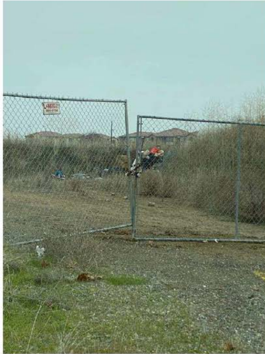
Shasta Reservoir, construction area temporary fencing
