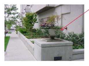
Flow-through planters are designed to treat and temporarily detain runoff without allowing seepage into the underlying soil. They typically receive runoff via downspouts leading from the roofs of adjacent buildings.
