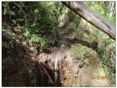
**Photo 7 (Site #4):** View of a road fill failure caused by diverted pond outflow. This erosion feature is located down the right road from the levee. Note the road prism is completely washed out.
