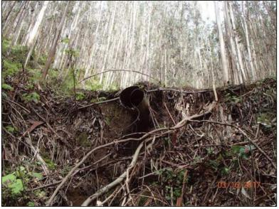
**Photo 21 (Site #9):** View of the perched culvert outlet at stream crossing Site #9. The culvert at this crossing is undersized and installed high and short in the fill with a 6ft drop at the outlet and subsequent outboard fill erosion.
