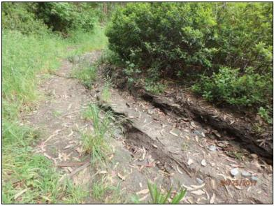
**Photo 23 (Site #16):** View of the left road approach to fill crossing Site #16. Diverted stream flow is actively eroding gullies down the left road from this stream crossing and delivering to a watercourse at Site #15.
