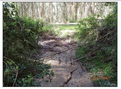
**Photo 13 (Site #39):** View looking downstream from the upstream extent of the of the failing stream crossing. Note the recently deposited sediments that have plugged the culvert inlets. The sediment is causing the stream flow to divert down the left road which is inducing a delivering fill failure.
