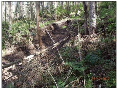
**Photo 11 (Site #19):** View of failing cutbank immediately upslope of the right edge of stream crossing Site #19. This cutbank failure delivers directly to the Class III stream in the axis of the crossing fill crossing.
