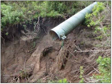
**Photo 16 (Site #40):** View of a section of disconnected culvert downspout at the top of an actively migrating headcut and gully below the paved Private Drive at Site #40. Oxidation exposed on the stake is indicative of the previous depth of burial prior to the episodic hillslope failure.
