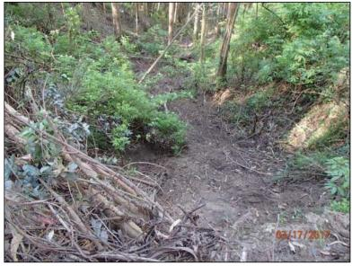
**Photo 12 (Site #19):** View of failing outboard fillslope, looking downslope at the fill failure deposits below the right hingeline of the fill crossing at Site #19. This photo was taken from the outboard edge of the road.
