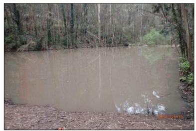
**Photo 4 (Site #4):** View of the on-stream pond located at Site #4 looking upstream from the left edge of the levee. Note the aggraded sediment at the upstream edge of the pond.
