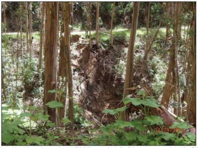
**Photo 14 (Site #39):** View of an outboard fill failure to the left of the stream crossing. The fill failure was induced by the diverted streamflow from the plugged stream crossing at Site #39 and excessive concentrated road surface runoff.
