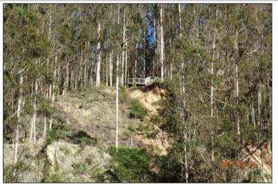
**Photo 33 (Lookout Vista):** View of the lookout deck and failing hillslope below the outermost footing. This photo was taken looking upslope from the base of the quarry floor.
