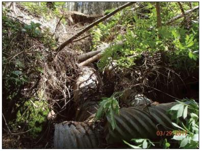
**Photo 15 (Site #39):** View looking upstream at the failing outboard fillslope of this plugged stream crossing. The photo was taken standing approximately 8ft downstream of the culvert outlets.
