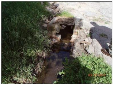
**Photo 24 (Site #23):** View of the outlet of the culvert at stream crossing Site #23 at the edge of the main parking lot. This culvert is undersized and stream flow avulses out of the drainage alignment and onto the parking lot surface.
