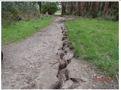
Photo 3 (Meadow Trail): View of active gully erosion along the Meadow trail. Combined diverted steam flow and concentrated road runoff are eroding the road surface along this native surfaced road.
