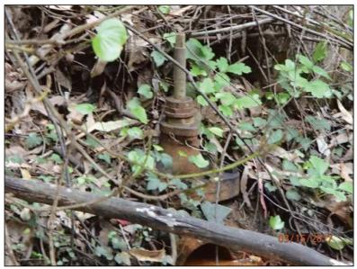
**Photo 8 (Site #4):** View of the seeping drainage valve at base of the dam fillslope in the axis of the valley downstream of pond.
