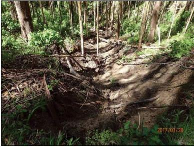
**Photo 26 (Site #31):** View of an outboard fill failure at Site #31 on the Vista Point Trail. Concentrated road run off had saturated the steep outboard fill and subsequently destabilized the fillslope leading to failure.
