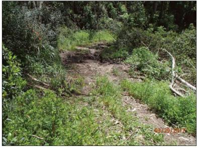
**Photo 22 (Site #16):** View of the fill crossing at Site #16 on the Dolphine Fire Road. Diverted stream flow is actively eroding gullies down the left road from this stream crossing.
