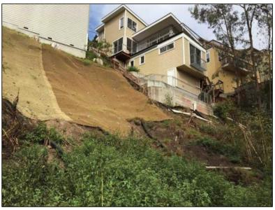
**Photo 20 (Site #41):** View of a hillslope failure and undermined residences upstream from Site #41. This area upslope extent of AOC 4 as discussed in the text of the report. This photo was taken from the outboard edge of the Fire Break Road upslope from the Upper Pond Legacy Road as shown on Map 2.
