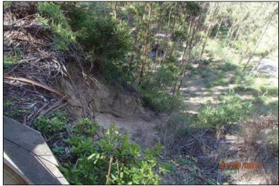
**Photo 34 (Lookout Vista):** View of the failing hillslope below the wooden lookout vista platform. The quarry cutslope is oversteep and is actively failing in multiple locations along the upper edge of the quarry area.
