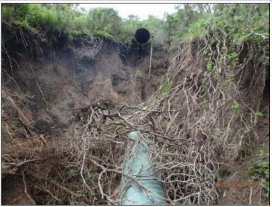
**Photo 17 (Site #40):** View looking upslope at the same disconnected downspout and active erosion as shown in the previous photo. The photo was taken from the base of the gully downslope of the headcut standing on top of one of the failed sections of culvert.
