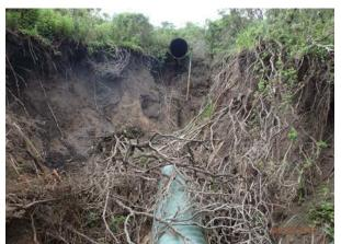
Damaged drainpipe causing gully erosion
