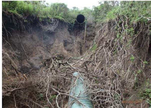
*Damaged drainpipe causing gully erosion*
