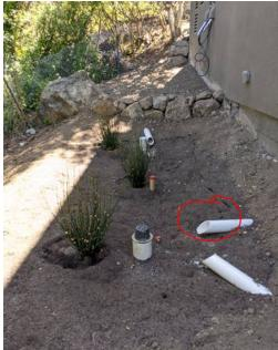
3. The lower discharge pipe on the big dissipator ended up much closer to the end of the dissipator then per plan. Please have your Civil Engineer confirm the amount/length of dissipation is adequate.
