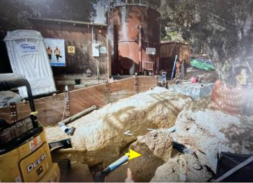
Photo 5. Northwest view of 2020 construction of water tank and booster pump at Cal Water Service Station 112 across from 742 Loma Ct. About 50 feet of new 6" diameter pressure line pipe was connected to the pre-existing line installed some
