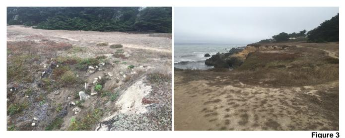
Photos of the bluff top showing concrete debris and fill at the top of an active landslide (left) and the variability in the bluff edge caused by gullies (right)
