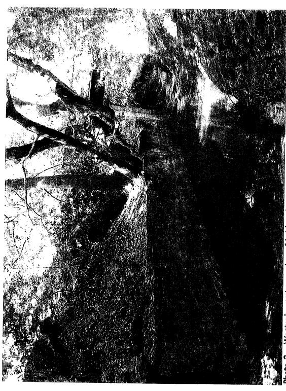
Resistant sandstone lines channel bottom at bridge crossing. Note local bank erosion in Photo 2 - Westerly, upstream view of bridge abutments and concrete wall on downstream side. distance and end-point erosion at downstream end of wall.
