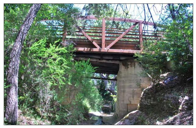
Figure 8: View east towards bridge and south bank – note stacked stone and concrete
