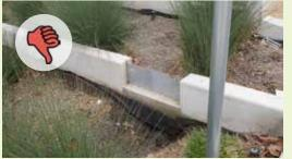
Without a hard splash pad, the soil downstream of this weir is experiencing significant erosion.
