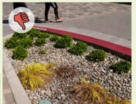
▲ Conversely, this stormwater curb extensions inlet rim is fixed at the finish grade of rock mulch leaving little opportunity for water retention.
