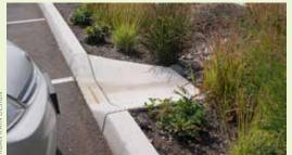
▲ Tapered concrete side walls conform to curb cuts with 45-degree chamfered edges.
