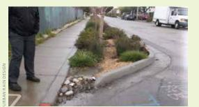
ock used to minimize erosion inhibits flow and creates sediment accumulation that is difficult to remove.
