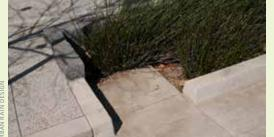
▲ A cleaned sediment forebay. The smooth, and hard surface allows for easy removal of sediment and debris.
