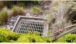
▲ Simply surrounding an existing flush inlet with raised bricks that use epoxy to seal gaps creates a simple raised weir effect and retains additional runoff
