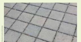
▲ The void space of pervious concrete should be free of sediment and debris by regular sweeping or blowing.
