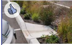
Condition: Curb cuts are properly graded and armored for erosion control.
