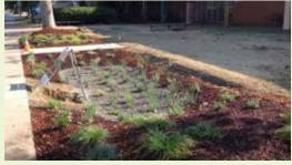
▲ The basin portion of this rain garden is mulched with pea gravel and the side slopes are covered with organic mulch.
