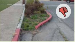
▲ This stormwater curb extension has no concrete forebay. Sediment builds up and blocks runoff from entering.
