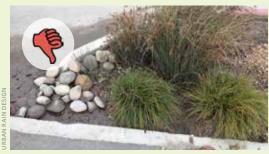
River rock used to minimize erosion creates pockets of sediment accumulation that is difficult to remove.
