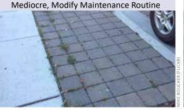
*Condition:* Some pervious paving joints are beginning to fill with sediment and debris slowing infiltration.
