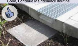
Condition: Splash pad at water flow point is adequately controlling erosion.
