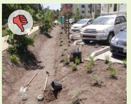
▲ This newly installed green infrastructure facility will have consistent problems with erosion control and plant health issues because of steep grading and side slope conditions.
