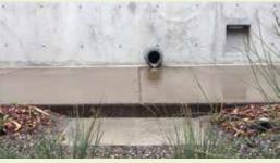
A concrete splash pad and pea gravel mulch at the spill point of water reduces the potential of erosion.
