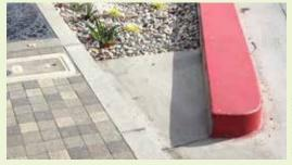
▲ While this is a good concrete pad, the elevation needs to be lowered at least 2 inches to allow for sediment capture.
