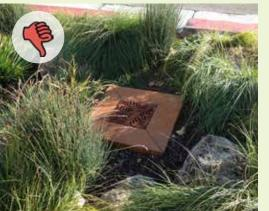
Conversely, this stormwater curb extension has no check dams and is graded to retain little stormwater. As a result, most of the runoff simply enters the inlet without any ponding of water.
