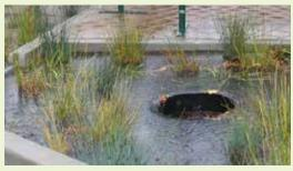
▲ This HDPE weir surrounds an inlet that is flush with the soil grade. The weir dictates the water level.
