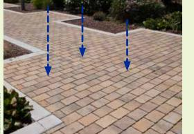
▲ This application of pervious pavers only has direct rainfall to manage. There is no impervious area runoff directed to it.
