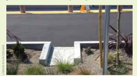
▲ This rain garden's curb cut is structured correctly and provides adequate drainage into the landscape
