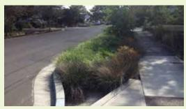
This stormwater curb extension has a concrete forebay that captures sediment that is removed regularly
