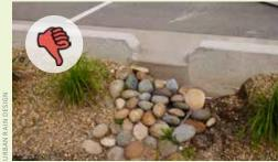
▲ Cobble placed at a curb cut entry does not allow for good erosion control or ease of water flow.
