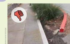
A stormwater curb extension curb cut full of sediment accumulation.
