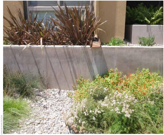
▲ A roof downspout uses a metal channel to direct roof stormwater into a planter area. It is critical that the planter maintains a rock mulch or concrete splash pad to dissipate the vertical energy of water spilling into the landscape area.
