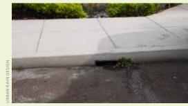
▲ This poorly designed and compromised curb cut should be replaced with a better design as part of maintenance.
