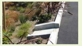
▲ This is a better curb cut option with hardscape walls and pea gravel mulch to control erosion.
