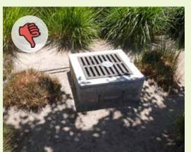
▲ This storm inlet's rim is placed at a fixed height of 8 inches. If this rain garden does not infiltrate at a reasonable rate, it is prone to the effects of prolonged standing water.
