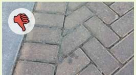
Sediment build-up within the joints of interlocking concrete pavers.
