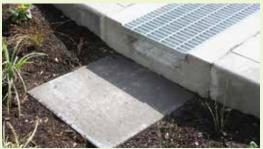
A concrete forebay at the street curb cut is placed lower than the gutter grade to disperse water flow.
