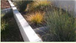
▲ This stormwater planter has several metal weirs placed along the flow path of water to encourage infiltration.
