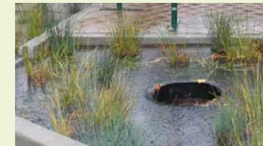
▲ This HDPE weir surrounds an inlet that is flush with the soil grade. The weir dictates the water level.
