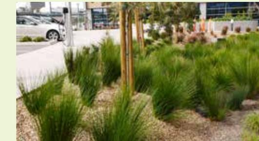
▲ Pea gravel mulch used on both the side slopes and wetted area of a vegetated swale prevents erosion.
