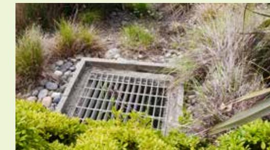
▲ Simply surrounding an existing flush inlet with raised bricks that use epoxy to seal gaps creates a simple raised weir effect and retains additional runoff.
