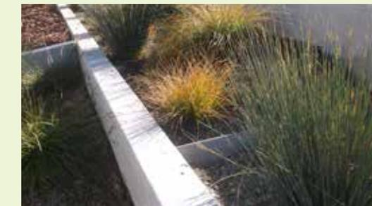
▲ This stormwater planter has several metal weirs placed along the flow path of water to encourage infiltration.
