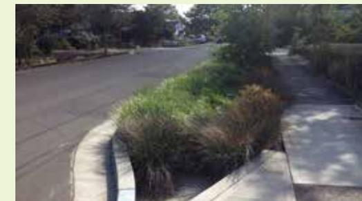
▲ This stormwater curb extension has a concrete forebay that captures sediment that is removed regularly.
