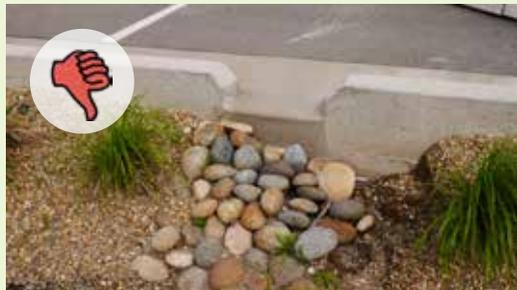
▲ Cobble placed at a curb cut entry does not allow for good erosion control or ease of water flow.
