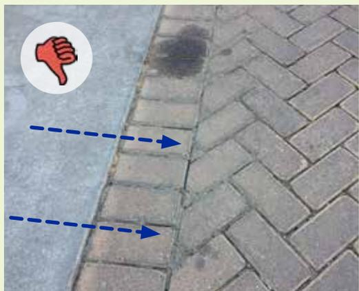
▲ Stormwater runoff and sediment from impervious area is flowing onto and constantly clogging the joint spaces of concrete interlocking pervious pavers.
