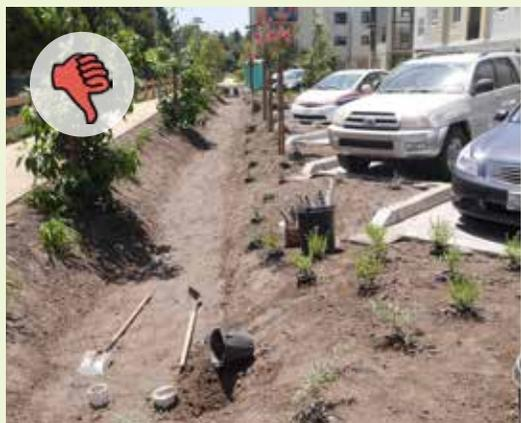
▲ This newly installed green infrastructure facility will have consistent problems with erosion control and plant health issues because of steep grading and side slope conditions.
