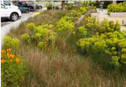
◀ Rain gardens function as soil and plant-based filtration devices that remove pollutants through a variety of physical, biological, and chemical treatment processes. These facilities normally consist of a ponding area, mulch layer, vegetation and biotreatment soil mix. Photo Credit: Urban Rain Design
