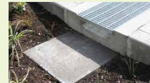
▲ A concrete forebay at the street curb cut is placed lower than the gutter grade to disperse water flow.
