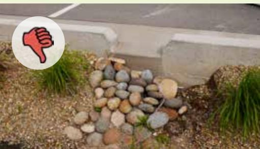
▲ It appears that the placement of rock prevents erosion, but runoff is moving around the rock and eroding soil.
