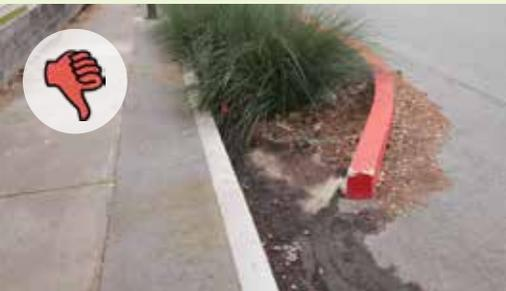
▲ A stormwater curb extension curb cut full of sediment accumulation.
