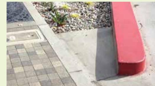
▲ While this is a good concrete pad, the elevation needs to be lowered at least 2 inches to allow for sediment capture.
