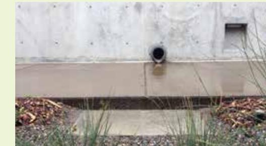
▲ A concrete splash pad and pea gravel mulch at the spill point of water reduces the potential of erosion.
