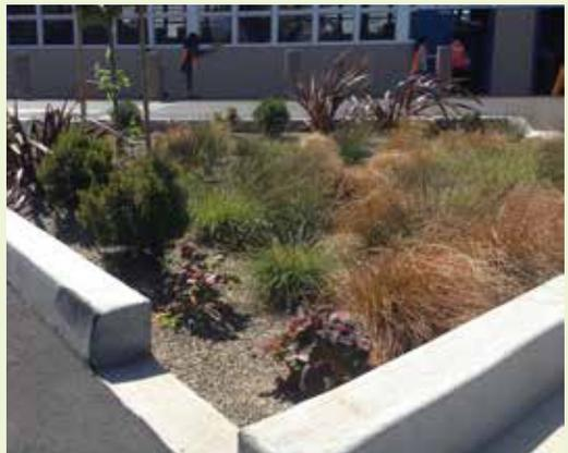
▲ This rain garden is graded very shallow to allow ponding of water, but it is not excessively deep or have steep side slopes. Ultimately this rain garden will perform better over time and will be easier to maintain.
