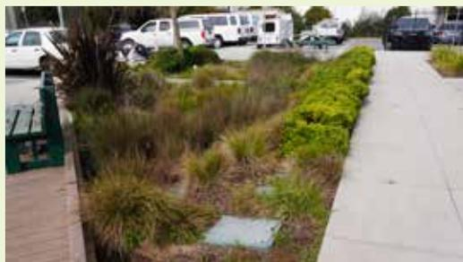
▲ This rain garden has about 70% plant coverage which is considered the minimum for functionality.
