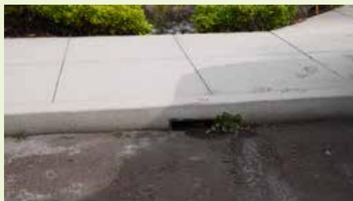
▲ This poorly designed and compromised curb cut should be replaced with a better design as part of maintenance.
