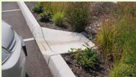
▲ Tapered concrete side walls conform to curb cuts with 45-degree chamfered edges.
