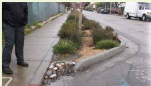
▲ River rock used to minimize erosion inhibits flow and creates sediment accumulation that is difficult to remove.
