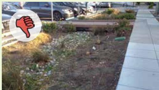
▲ This vegetated swale contains less than 70% coverage of plant material and needs additional plant material added.
