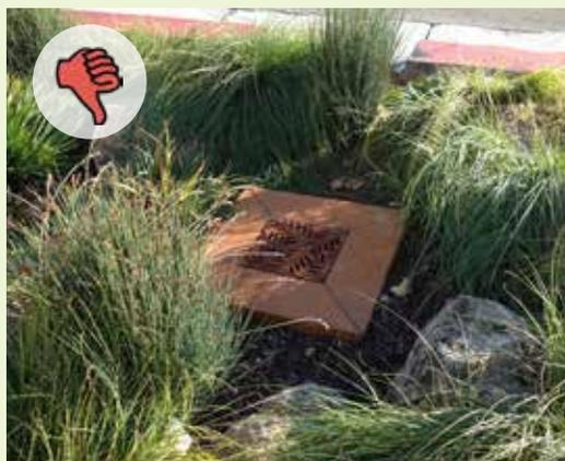
▲ Conversely, this stormwater curb extension has no check dams and is graded to retain little stormwater. As a result, most of the runoff simply enters the inlet without any ponding of water.
