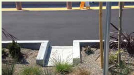
▲ This rain garden's curb cut is structured correctly and provides adequate drainage into the landscape.
