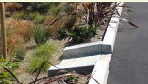
▲ This is a better curb cut option with hardscape walls and pea gravel mulch to control erosion.
