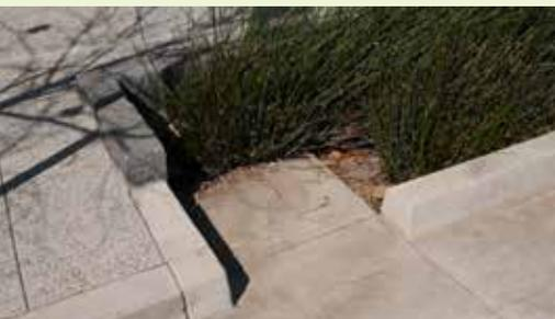
▲ A cleaned sediment forebay. The smooth, and hard surface allows for easy removal of sediment and debris.
