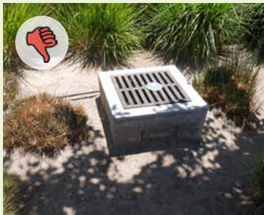
▲ This storm inlet's rim is placed at a fixed height of 8 inches. If this rain garden does not infiltrate at a reasonable rate, it is prone to the effects of prolonged standing water.
