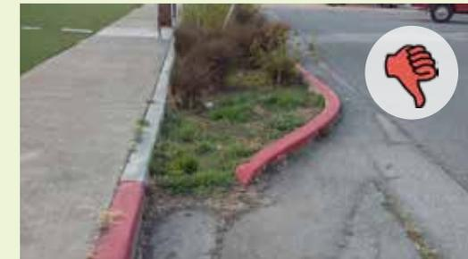
▲ This stormwater curb extension has no concrete forebay. Sediment builds up and blocks runoff from entering.
