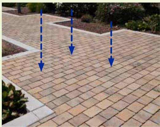
▲ This application of pervious pavers only has direct rainfall to manage. There is no impervious area runoff directed to it.
