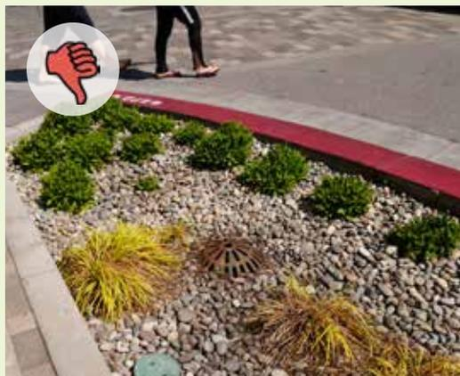
▲ Conversely, this stormwater curb extensions inlet rim is fixed at the finish grade of rock mulch leaving little opportunity for water retention.
