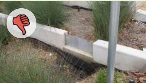
▲ Without a hard splash pad, the soil downstream of this weir is experiencing significant erosion.
