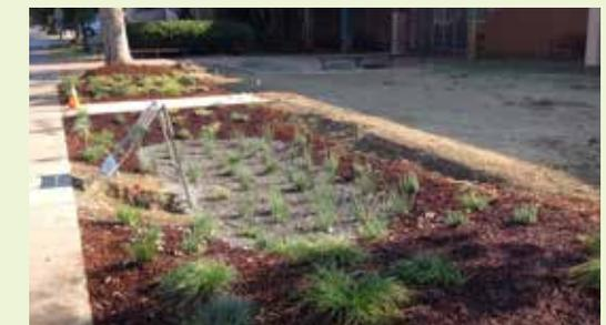
▲ The basin portion of this rain garden is mulched with pea gravel and the side slopes are covered with organic mulch.
