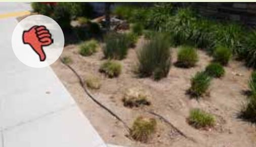
▲ A rain garden without regular mulch replacement results in plant desiccation and exposed drip irrigation lines.
