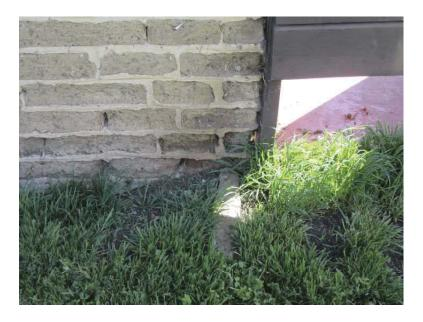
Photo 8. Restroom D showing eroded adobe units at base of wall. Minor regrading to direct the water away from the building will reduce future maintenance.
