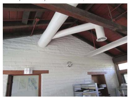
Photo 2. Interior adobe wall showing the gable above the bond beam. Gables act as parapets, which topple in earthquakes. They need to be attached to the roof structure. Roof framing and trusses chords can be seen.
