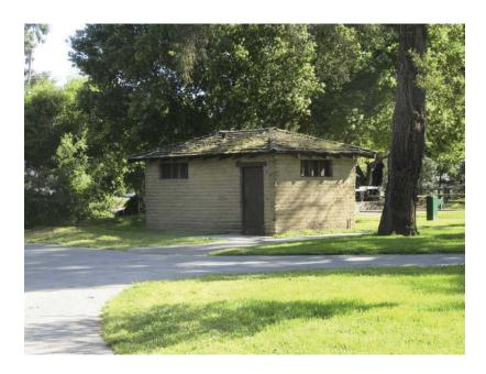
Photo 5. Maintenance Building near north end of site. Hip roof with shakes is part of the rustic style used by the WPA.
