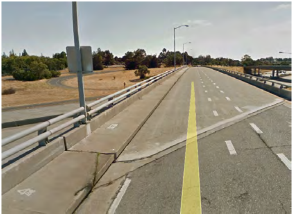
North Sand Hill Road overcrossing and sidewalk
