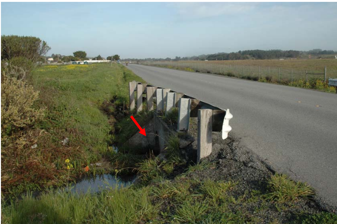
Photograph 2. Twin concrete culverts (44" diameter) under Airport Road at the eastern perimeter of the Big Wave Project Site. Large culverts carry storm water runoff under Airport Street to the Big Wave Project Site.
