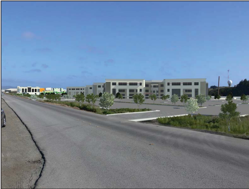
View 1.A: Looking south across the project site from Airport St with immature landscaping.
