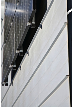
1. standing seam roofing
