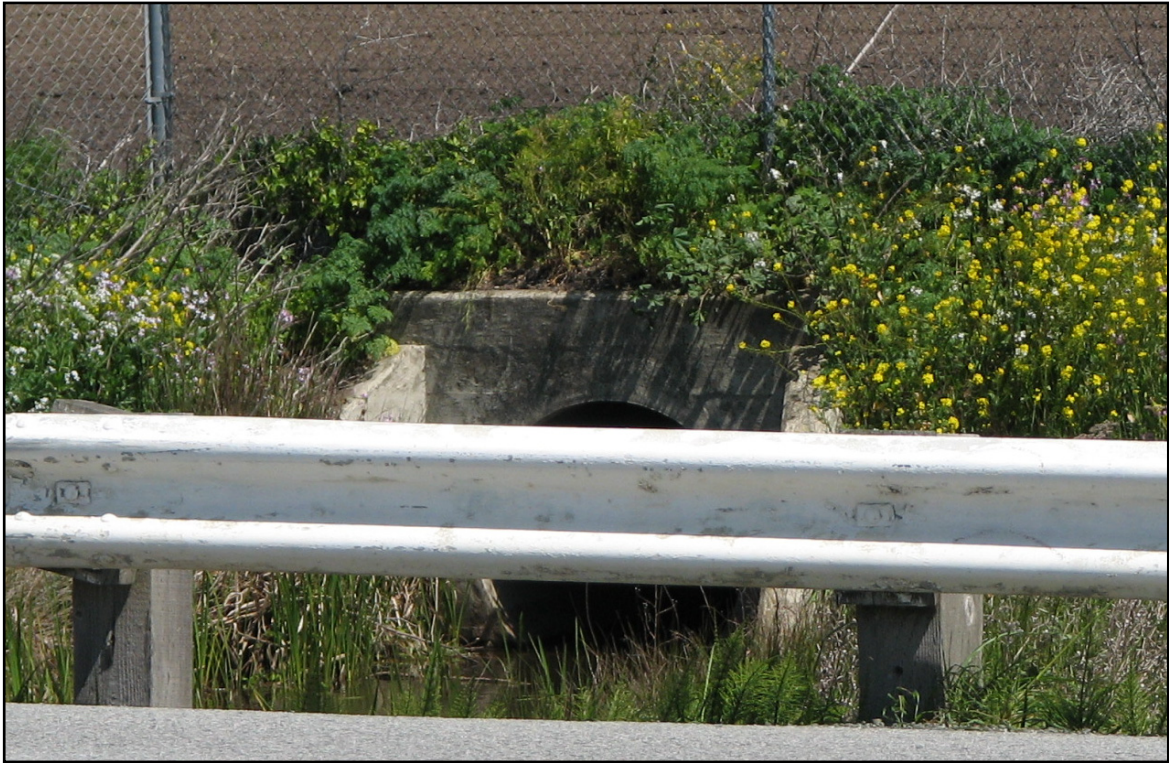
Surface water drainage culverts up stream of site.
