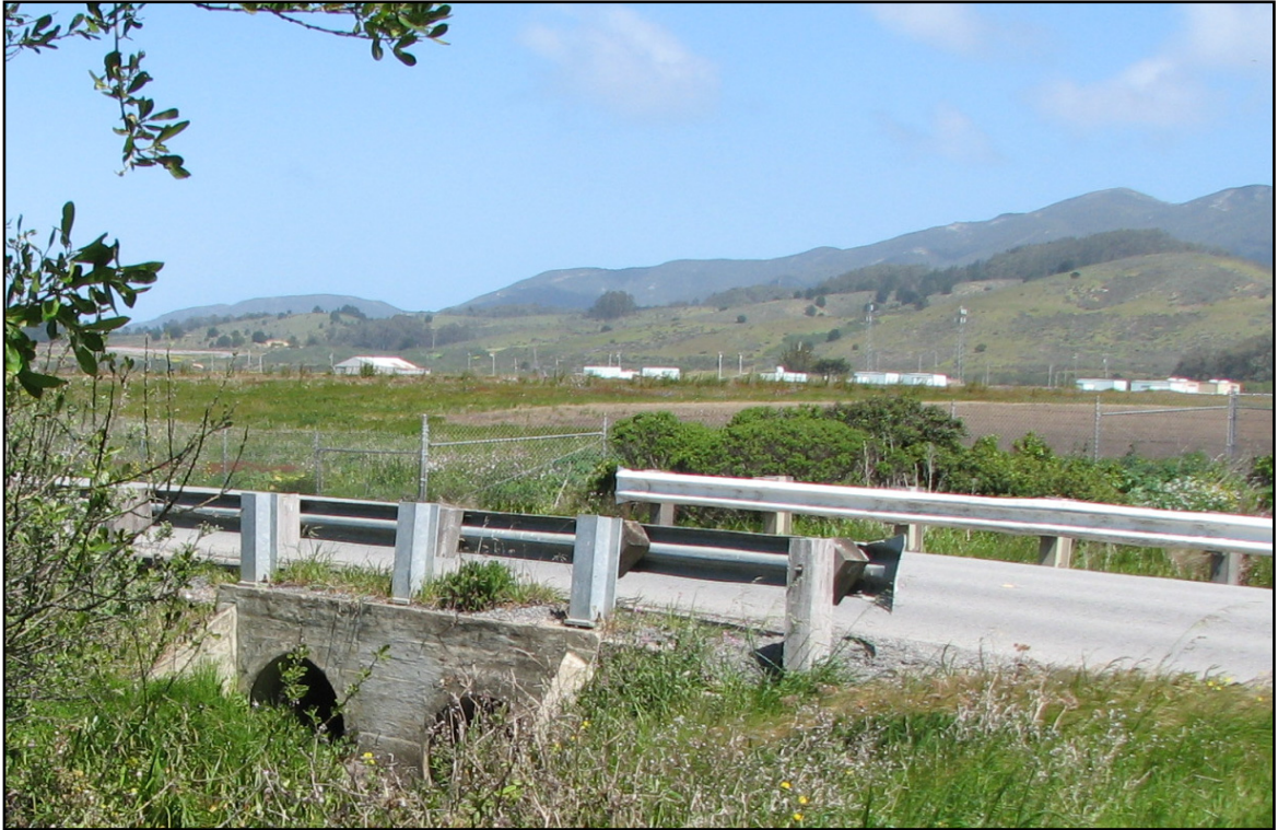
Surface water drainage culverts on site.
