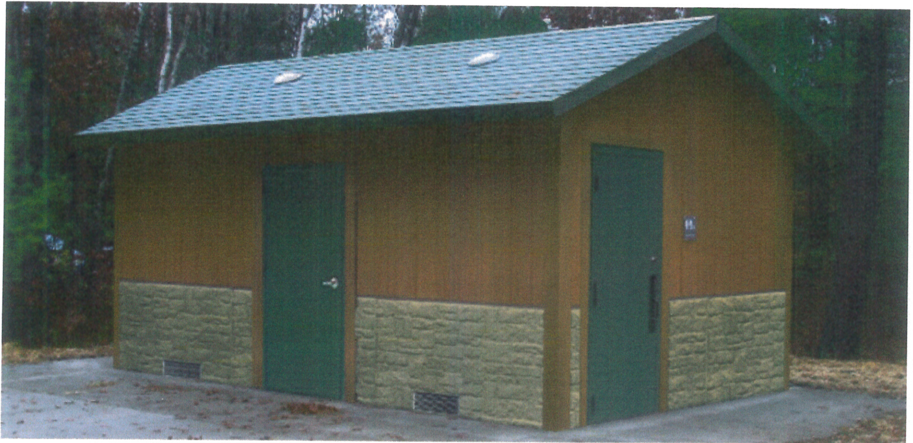
Precast/Preassembled Reinforced Concrete Bathroom
